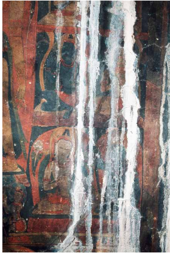
226 Detail of the water damage on the north-western wall. CL 2003.
