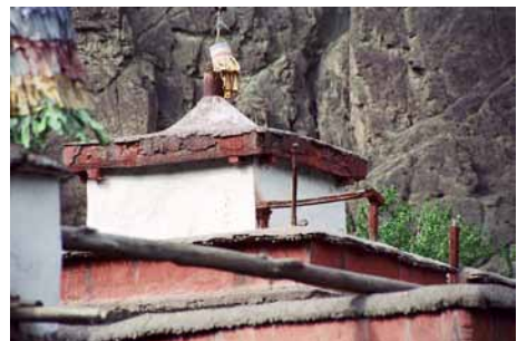
56 Detail of lantern roof eaves at the Sumtsek. HN 2003.
