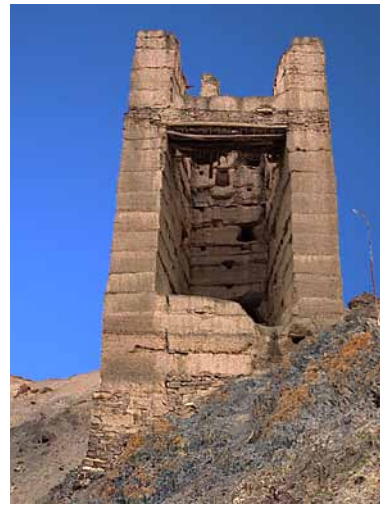
27 North-western view of the earthen tower (I). HN 1998.
