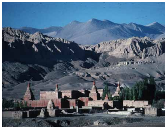
171 The mandala temple in Tholing prior to its restoration. CL 1993.
