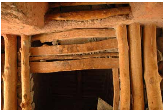
257 Ceiling construction inside the gateway chorten. DL 2009.
