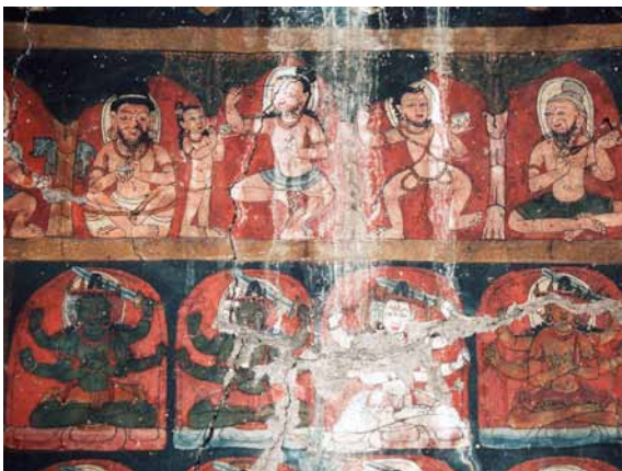
227 Cracking and water damage on the south-western left side wall. CL 2003.
