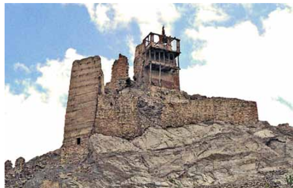
24 The front side of the central tower with the three-storied wooden gallery. HN 2003.
