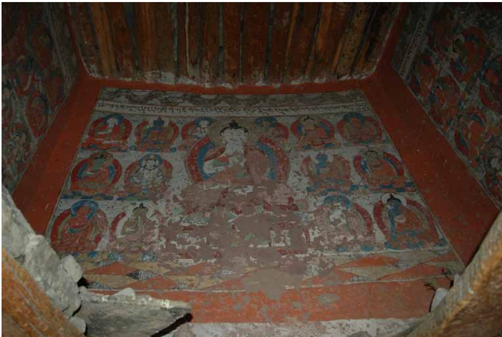
260 North-eastern (above) and south-eastern interior walls of the gateway chorten. DL 2009.
