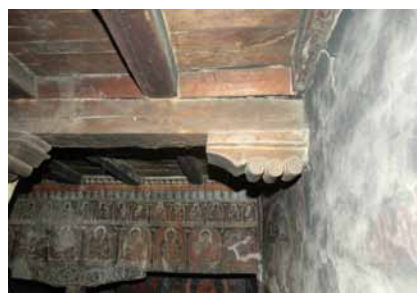
82 Opening to the lantern seen from below. CL 2003.
