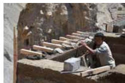
16 Eave construction. CA 2011.
