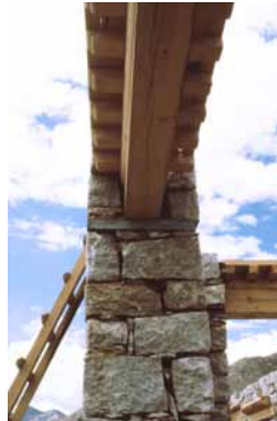
13 Lintel with crossbars, covered with boards. HN 1987.
