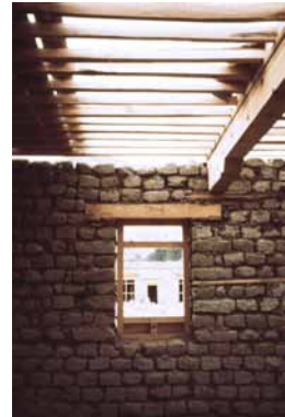
14 Cross beams resting on wall brackets. HN 1987.
