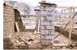
12 Brick wall and supporting stone pillar. HN 1987.
