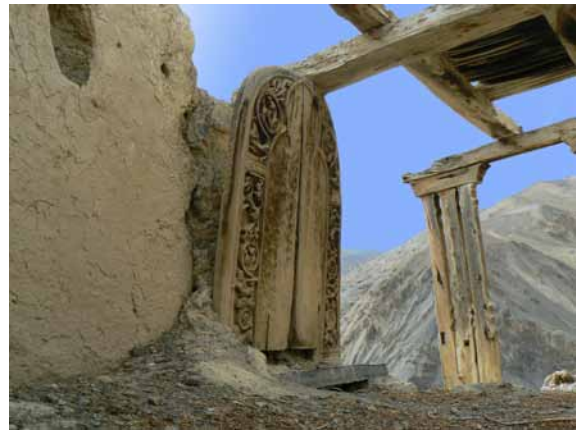
30 The upper floor of the the tower's fragile balcony showing the location of a carved nimbus placed on a stone slab. Heinrich Pöll 2008.
