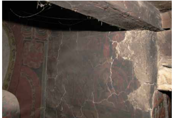
210 North-western niche with former repairs beside the lion corbel. DL 2009.
