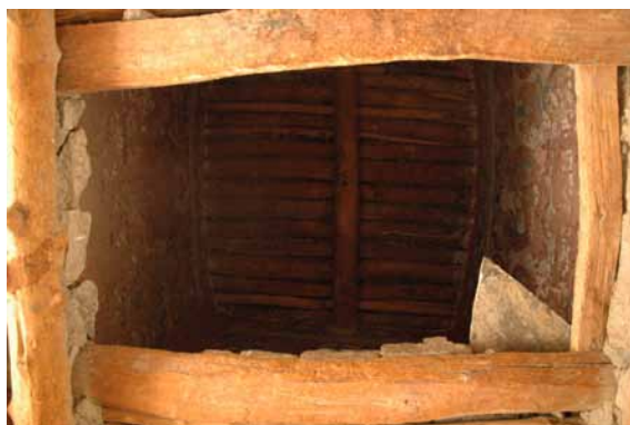
258 Opening to the painted chamber inside the chorten. DL 2009.
