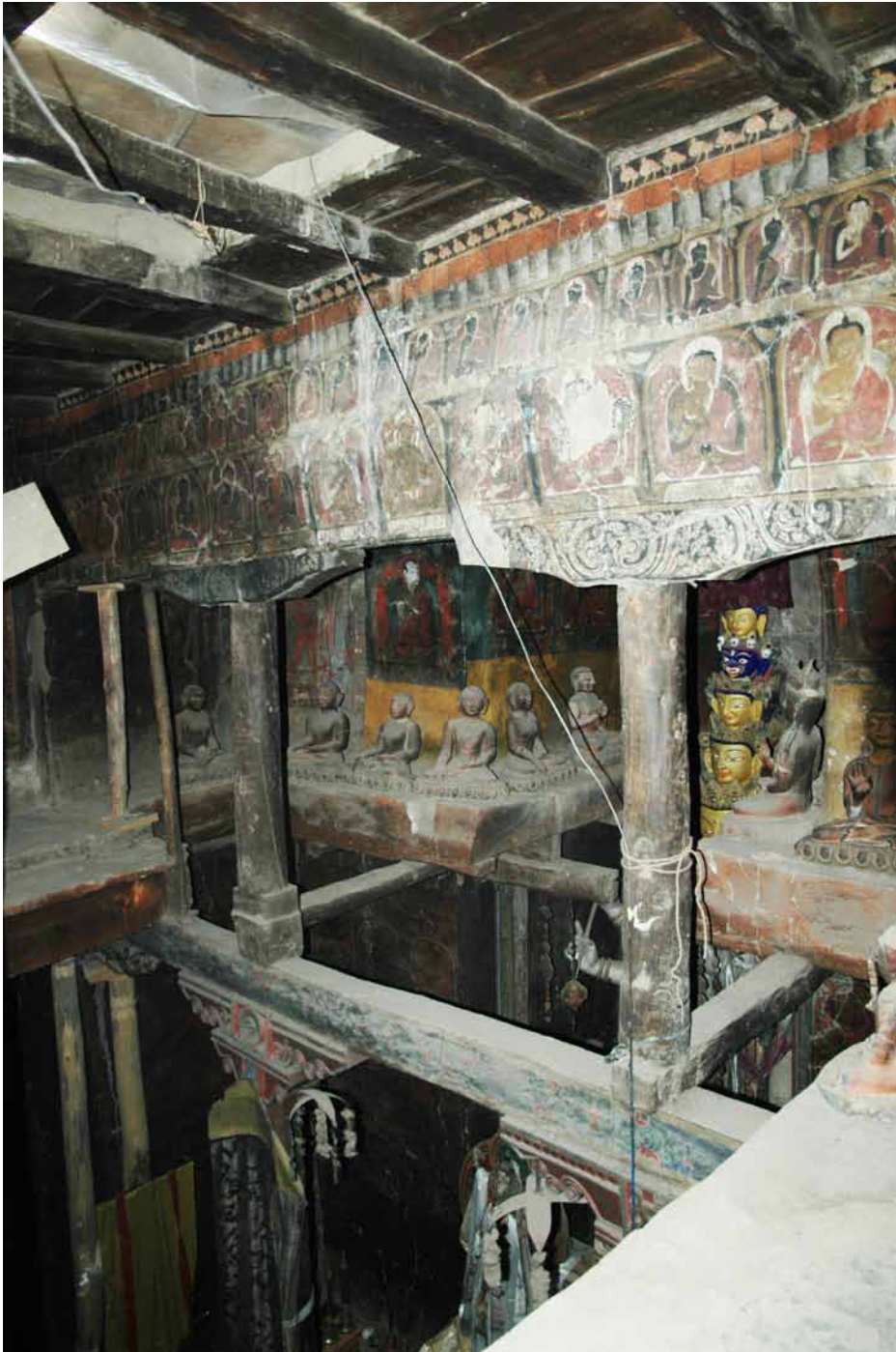
237 General view of the main apse area. DL 2009.
