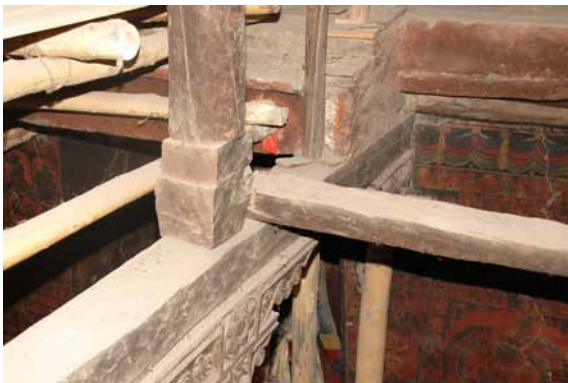
80 The base of the column on the south-east side. DL 2009.
