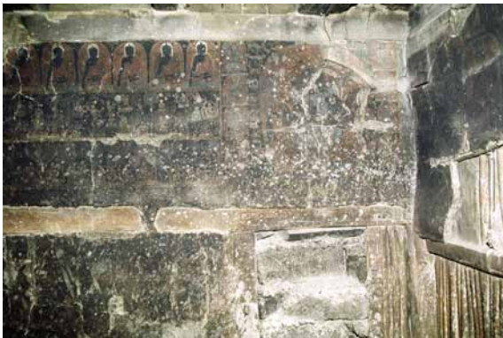
92 Walled entrance opening on the north-eastern wall. CL1998.
