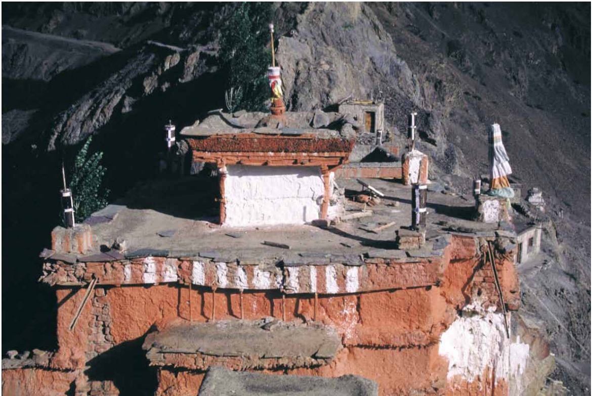
232 General view of the roof area. The eaves of the lantern, the main roof, the main apse, and the side niches are all shaped differently, HN 1998.
