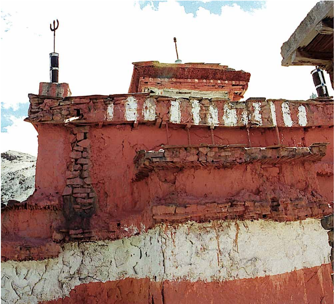
197 North-western view of the temple showing parts of the natural stone masonry in the area of the water damage on the facade, caused by the waterspout. HN 1998.
