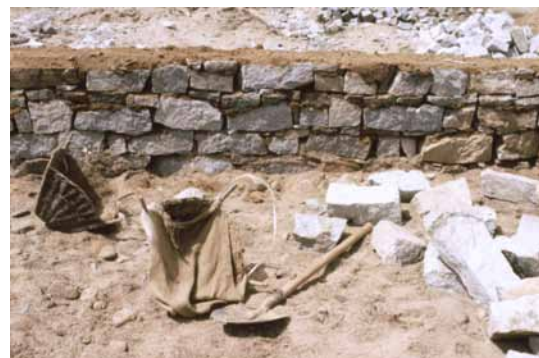
08 Stone masonry as a basis of the wall. HN 1987.
