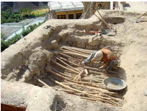
223 Broken rods from the flat roof construction over the false panelled ceiling of the main apse. Roland Pabel 2008.
