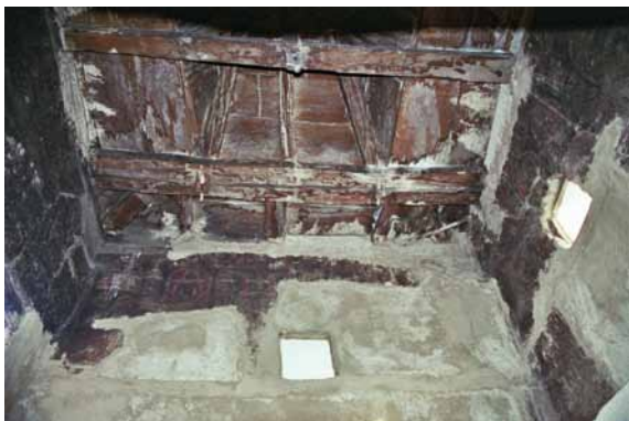
94 The hipped roof above the lantern. HN 2004.
