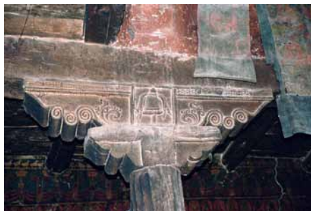
76 Painted capital below the main beam. DL 2009.
