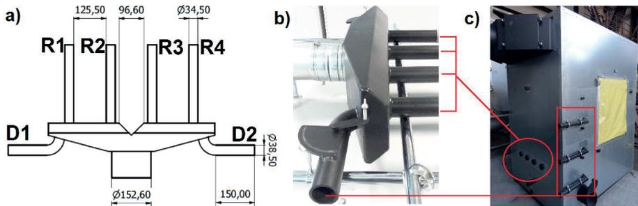
Figure 1. Projections of the studied air manifold (top view): (a) picture of the actual air manifold and (b) the location of the connectors in the boiler, (c) primary air nozzles marked with a circle and one (on the left side wall) of the two series of secondary air nozzles, marked with a rectangle.
