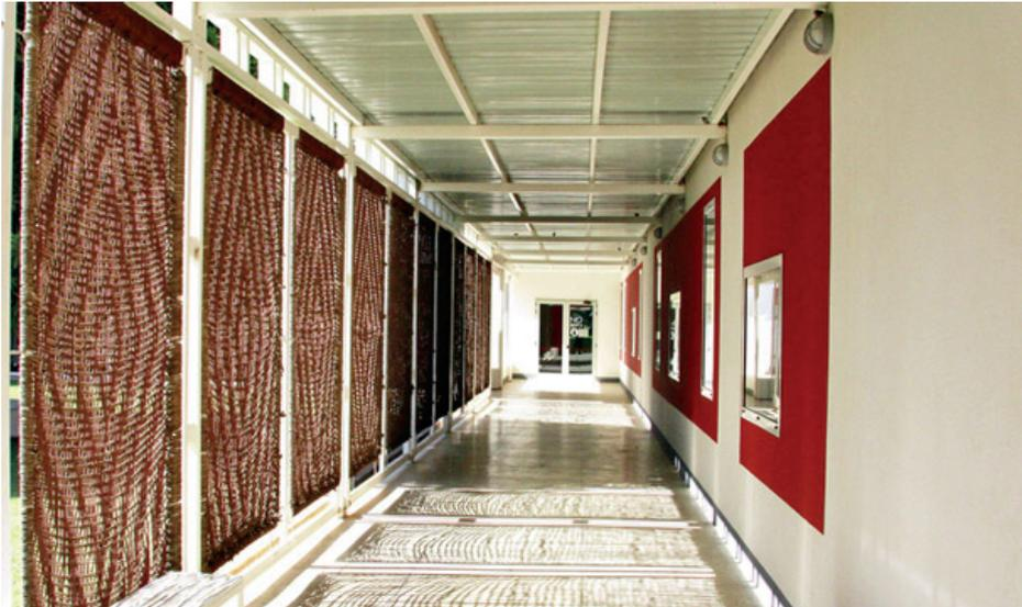
Fig. 2: A detail of the porticos of the Salam Centre with the twined vegetal panels on the left and the small double-screen windows on the right (photo by *Emergency* NGO<sup>6</sup>)
