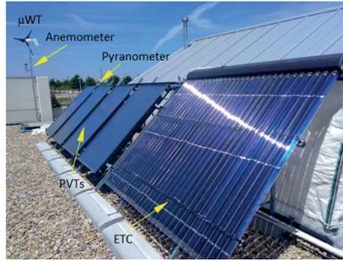
Figure 2.1: Detail of the  $\mu$ WT, PVTs and ETC of the pilot unit.
