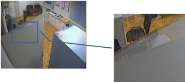
Figure 5. Bad placement of the surveillance camera—when the door is open, it occludes a large portion of the room, including the vault—the most important object in the room from a security viewpoint.
