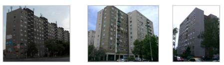
Three typical prefabricated reinforced concrete large-panel buildings in Hungary: building codes in order: terraced panel building, A10 and Kf10.
