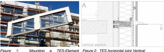
1: **TES-Element** Figure 2: TES horizontal joint Vertical Figure Mounting [gumpp&maier]
