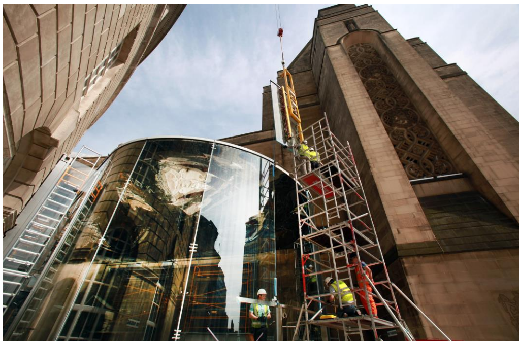
Figure 1: Glazed link building when the last glass element was installed.
