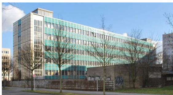
Figure 1: Type Leipzig, curtain wall façade, weather shell made of enameled steel sheets, Berlin Siegfriedstraße.
