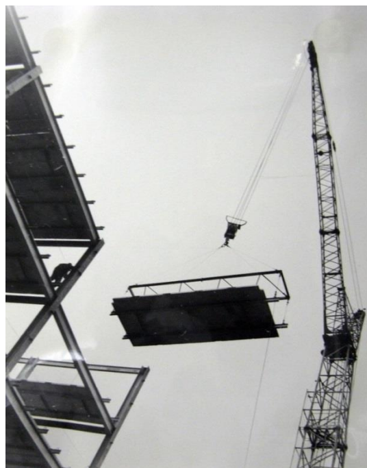
Figure 4: Prefabricated composite-steel deck floors.
