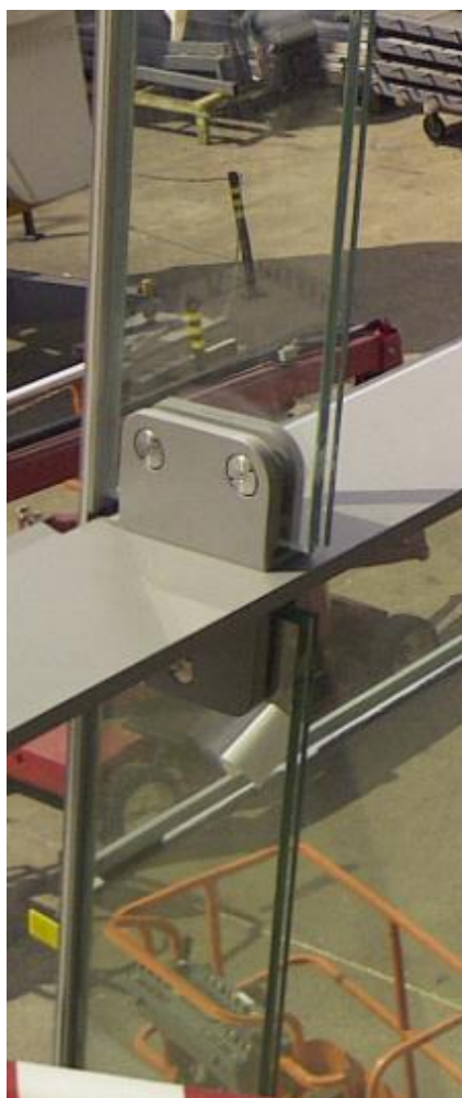
Figure 5: Glass fin solution with intermediate steel flat bar (left), project rendering Columbia University Medical Center © Diller Scofidio + Renfro (right)
