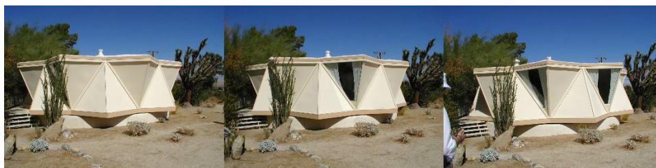
Figure 2. D'Angelo House, Snow Creek, Palms Spring. A rotating structure for minimizing the solar impact (picture courtesy of B.Sommer).
