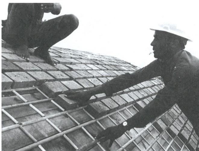
Figure 1: Arrangement of bricks on formwork [5]
