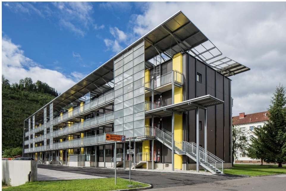
Figure 6: Renovation of the Johann Böhm apartment block after completion
