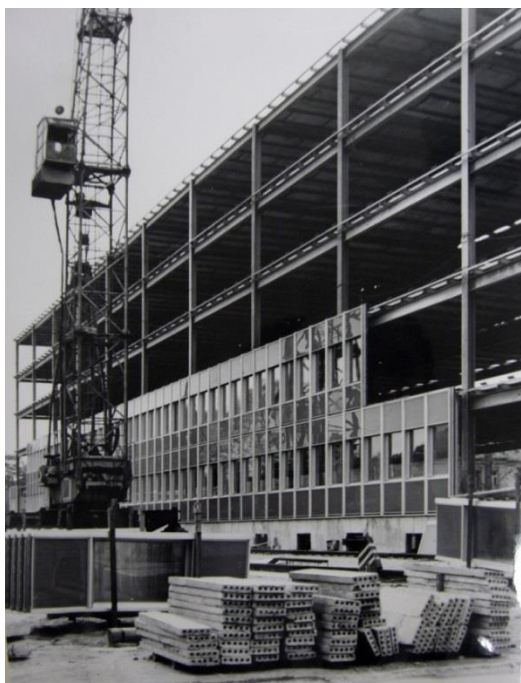
Figure 3: Installation of the unitized façade.
