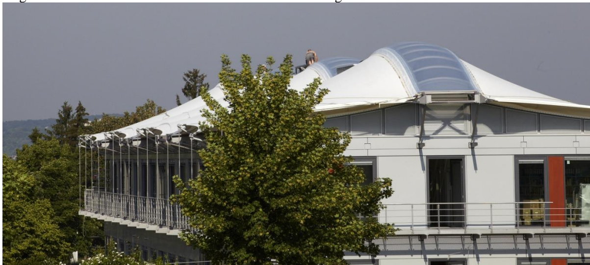
Figure 1: Energy Efficiency Center viewed from south-east. Clearly visible is the textile roof with translucent PTFE-glass membranes and partially transparent ETFE films.
