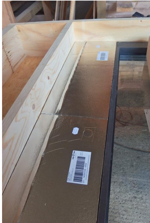
Figure 3: Prototyping - Left: Model for development studies (Thermowood, cement based boards, venetian blinds integrated). Right: Placing of vacuum insulation boards into full scale prototype
