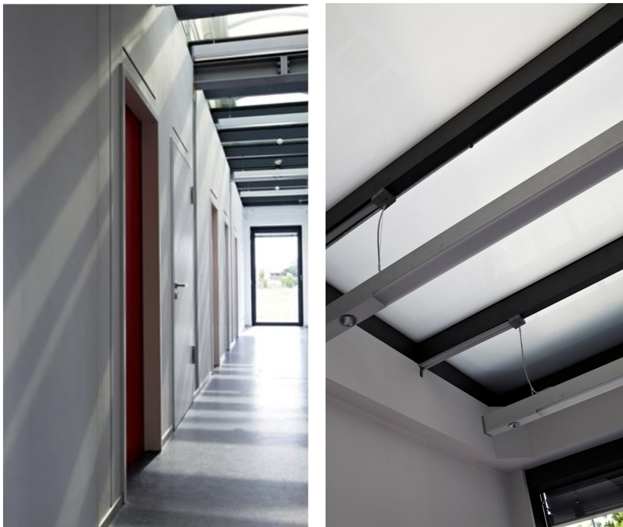
Figure 3: Corridor in the 1st floor in east-to-west direction illuminated by daylight (left); Translucent aerogel glazing in the stairways (right).
