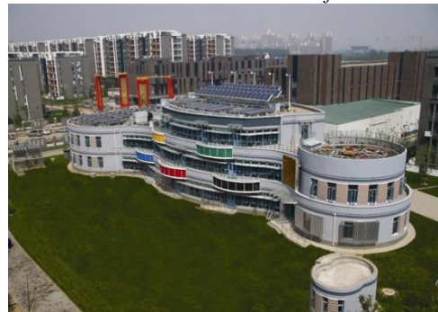
Micro energy consumption Kindergarten of Beijing
