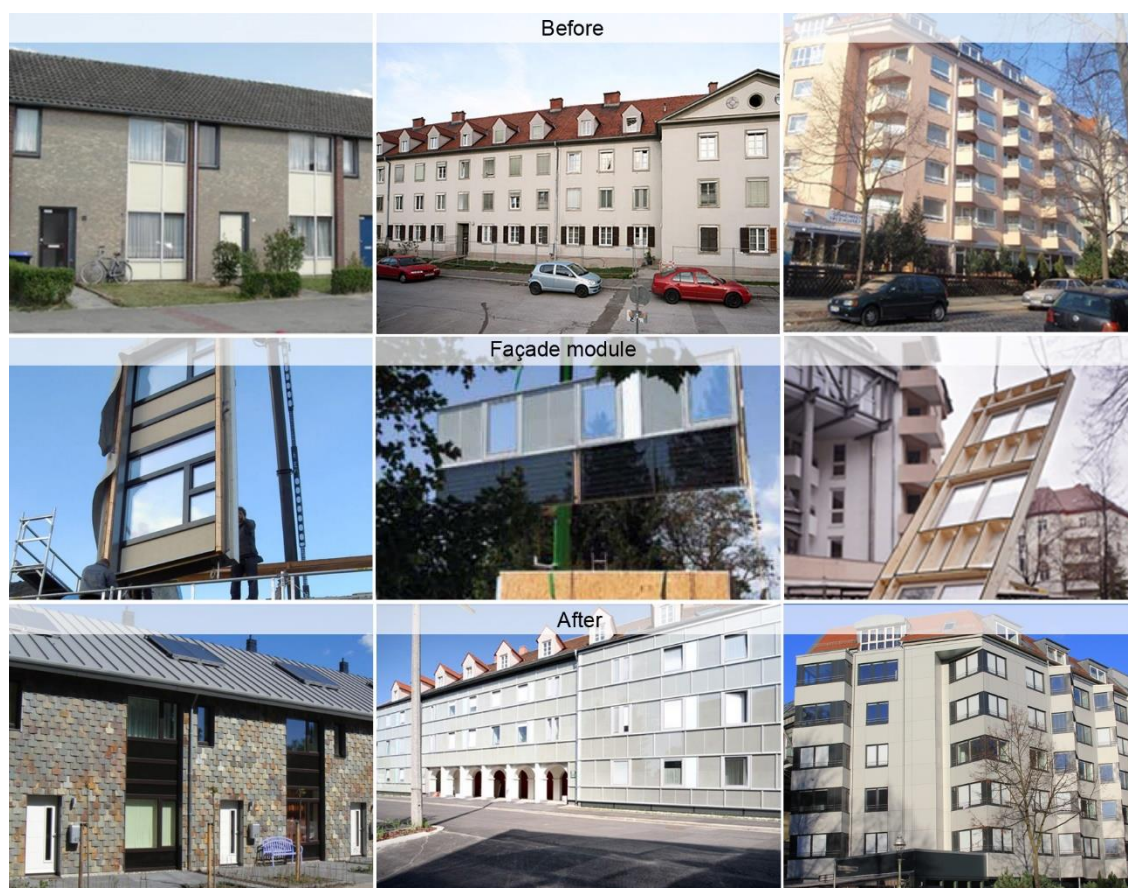
Figure 8. Some exemplary cases used to illustrate the guidelines; (left) terraced houses retrofitted with closed TES modules (Roosendaal, NL), (middle) terraced houses retrofitted with a solar façade system (Graz, AUT) and (right) an apartment block retrofitted with open TES modules (Berlin, GE)
