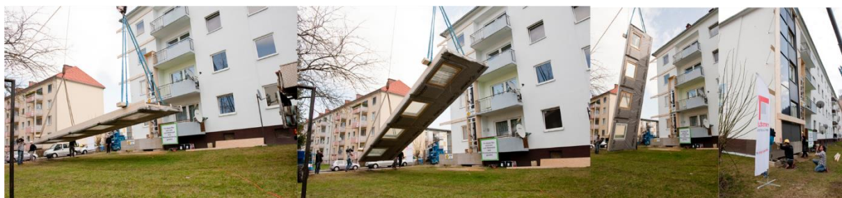
Figure 3: Attachment of the façade modules
