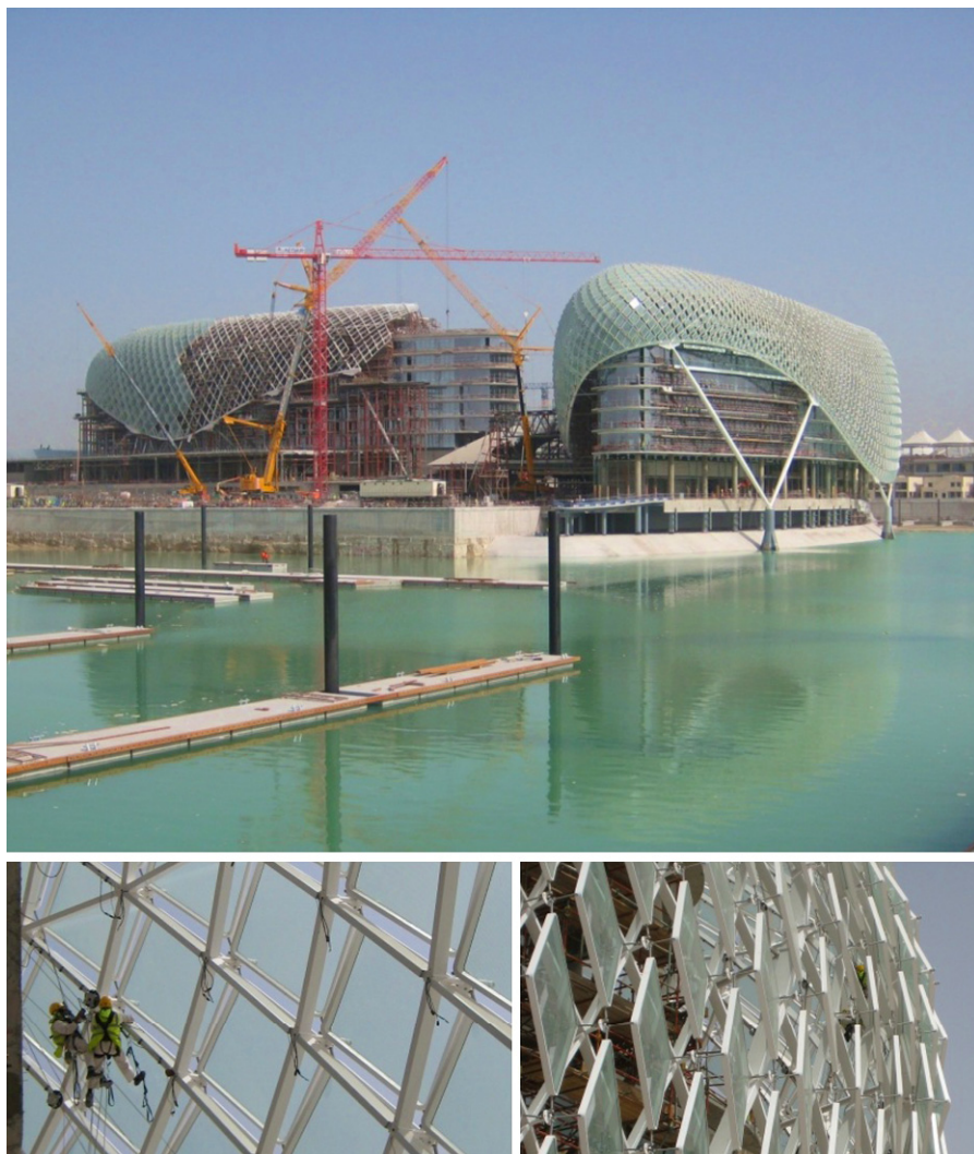
Fig. 4 Yas Island Hotel during construction. At bottom left one can see a detail of the outer skin which exhibits torsion-free nodes (images courtesy Waagner-Biro Stahlbau).
