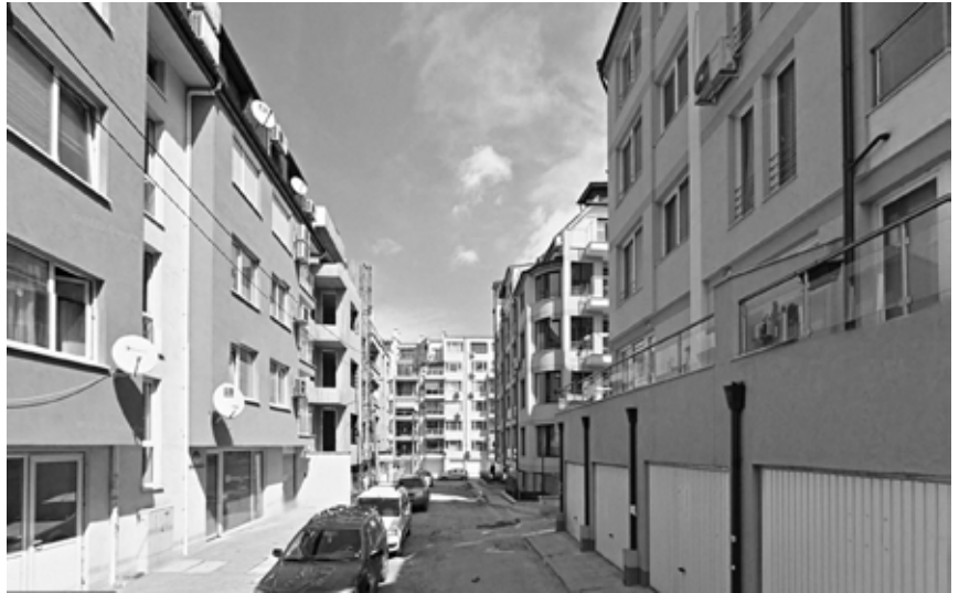
Fig. 6 New housing construction with dubious quality in the inner city neighbourhood Reduta. (Google Earth)
