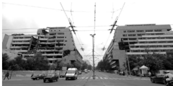
Fig. 6 The complex of the General Staff after the destruction during the NATO intervention, 1999. (Archive Samardžić)
