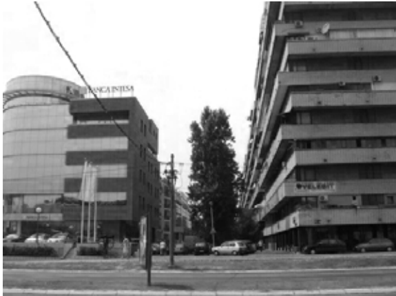
Fig. 12 New structures in Block 21 built during the last decade. (Đukić)
