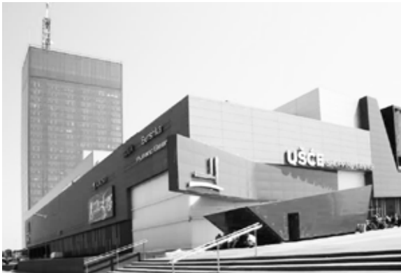
Fig. 10 Palace Ušće after the reconstruction. (Đukić)
