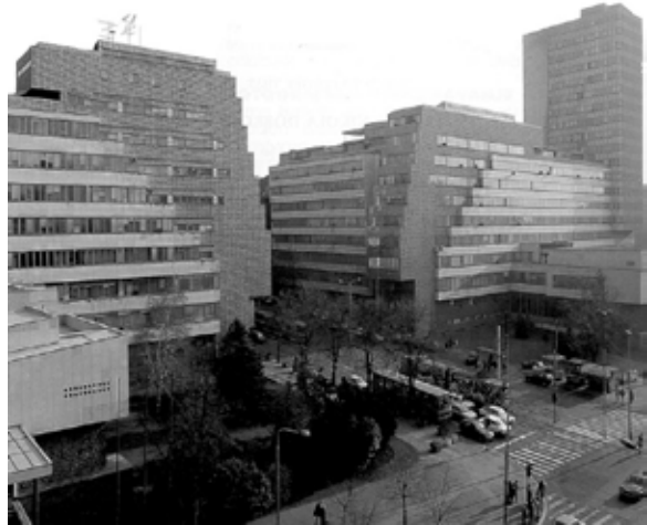
Fig. 5 The newly accomplished building complex of the General Staff. (Archive Samardžić)
