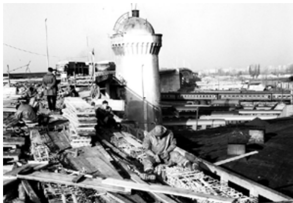
Fig. 2 The construction of the “Gazela” Bridge. (Archive Samardžić)
