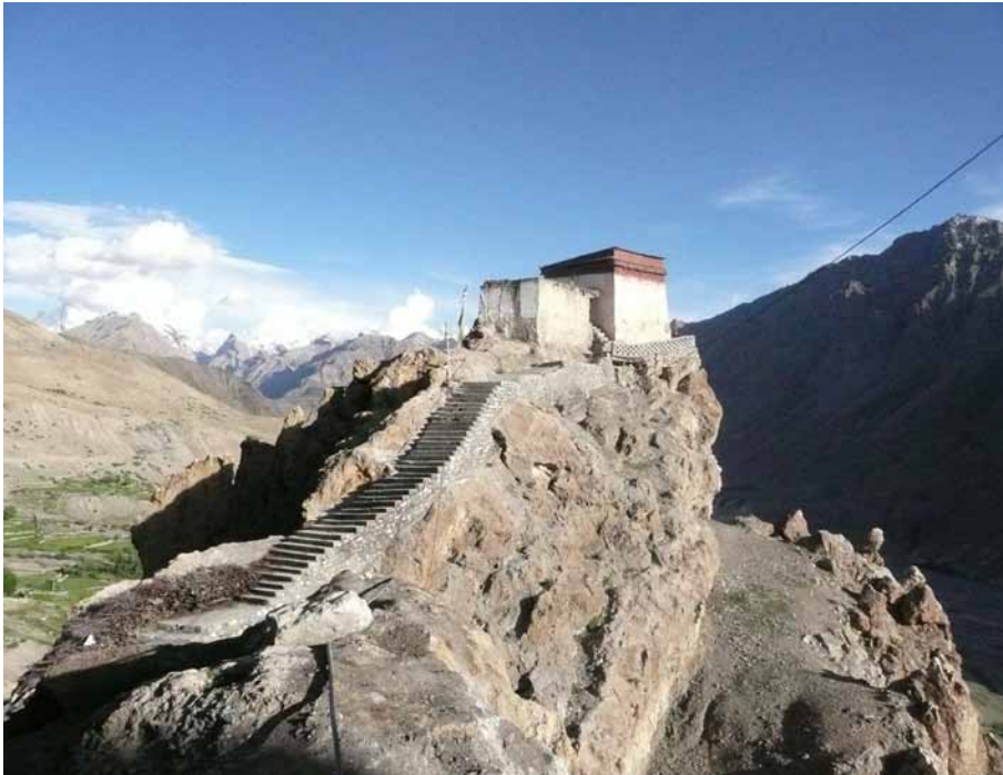
114 View from the north-west. CA 2010.
