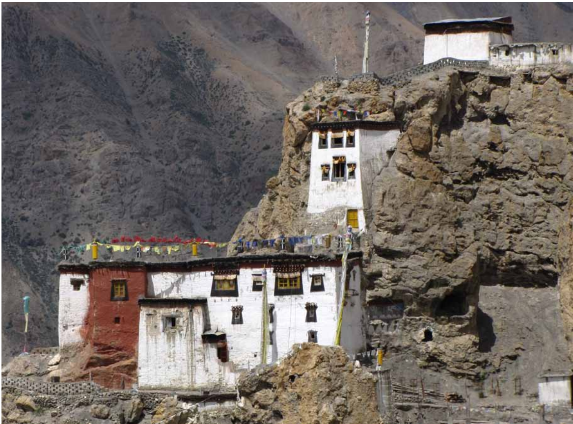
241 Eastern view of the tower above the roof of the monastery's main building. LN 2010.
