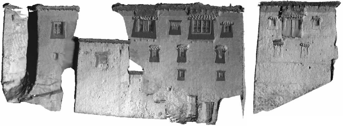
34 Eastern and northern facade of the monastery's main building digital 3D measurement. K&S TU Graz 2011.
