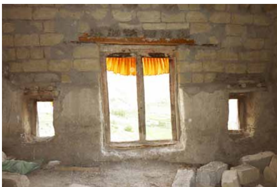
112 Windows of the south-eastern facade in the first floor. HN 2010
