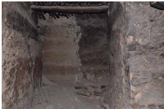
79 Walled up passageway to the adjoining assembly hall. CA 2011.
