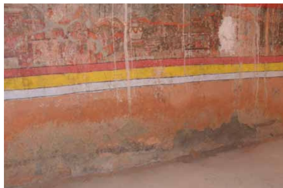
287 Dampening in the bottom area inside the upper temple. CA 2011.
