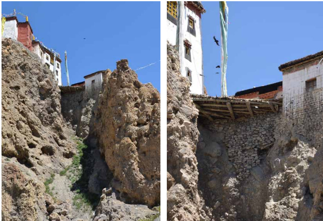
232 Erosion gully along eastern side of the ancient monastery and southern side of the kitchen (note partial undermining of block-mortar work in the erosion headwall). CA 2011.
