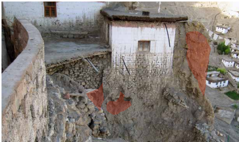
257 Underpin foundation elements along southern side of the kitchen. K&S 2011.
