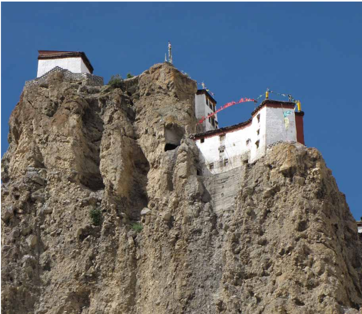
172 The upper temple above the main monastery building. View from south-west. LN 2010.
