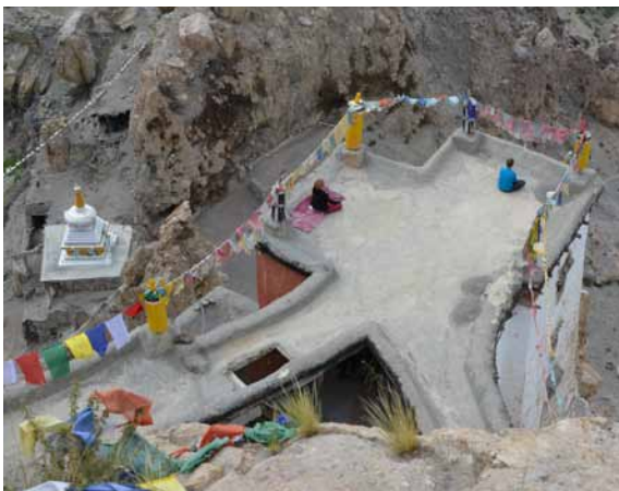
111 Roof area of the main building. CA 2011.
