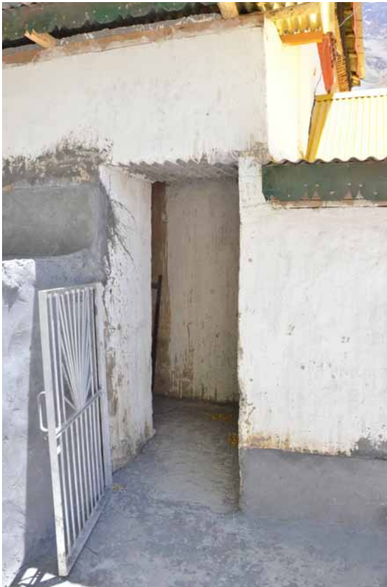
346 New entrance to the ambulatory on the northern side. CA 2011.
