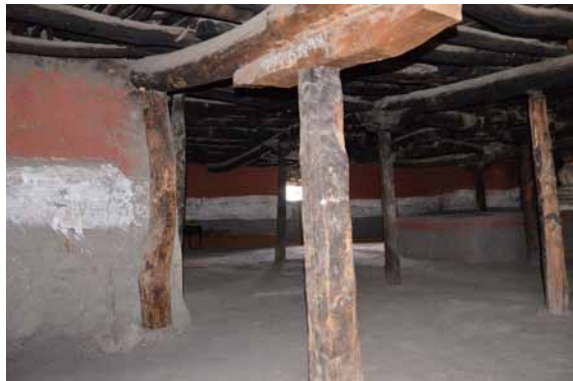
72 North-eastern corner of the room next to the east facade. CA 2011.
