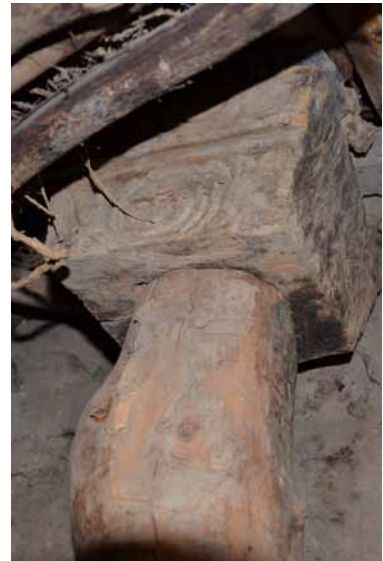
66 Carved column capital in room 4. CA 2011.
