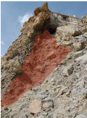
256 Shotcrete protection and underpinning along northern side of museum. K&S 2011.
