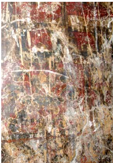
305 Losses of paint layers, thinned painted surface and deposits. G&S 2011.
