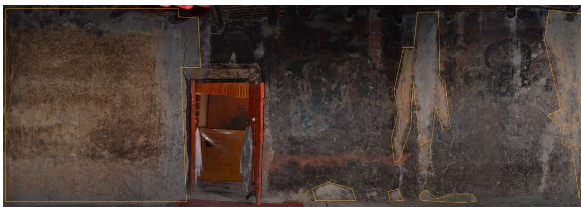
291 Map of the assembly hall. The eastern wall with the extent of undecorated plaster, repair and recoated surfaces indicated. University of Applied Arts Vienna 2011.
