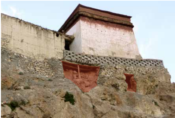
260 Underpin foundation elements along western side of the upper temple. CA 2011.
