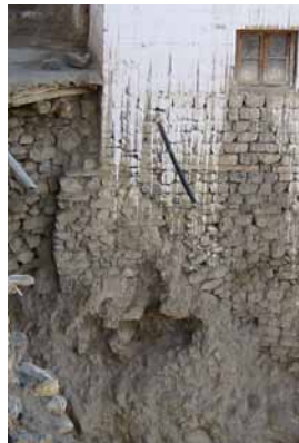
239 Partial undermining of block/mortar slope repair and foundation along southern side of the kitchen (note drain pipes). K&S 2011.
