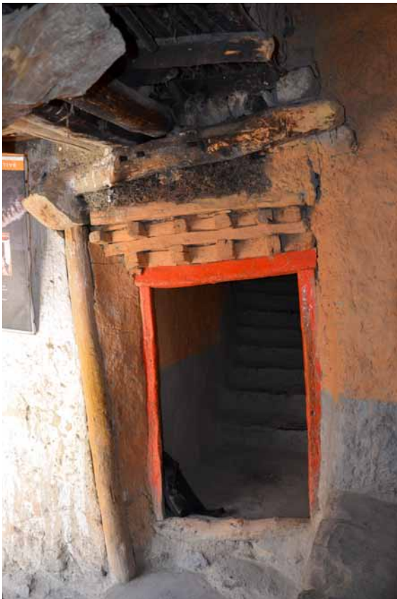
42 Construction of the old door opening to the interior stairway. CA 2011.
