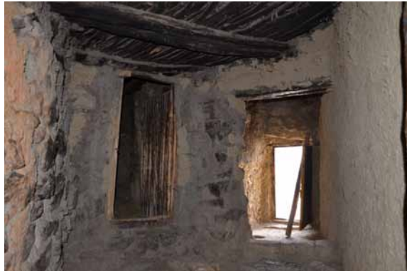
59 Passage with access to the terrace on the south-western side. CA 2011.
