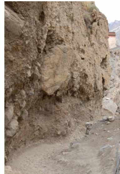
229 Differential erosion of block and matrix components, leading to the undermining and loosening of large block components. K&S 2011.
