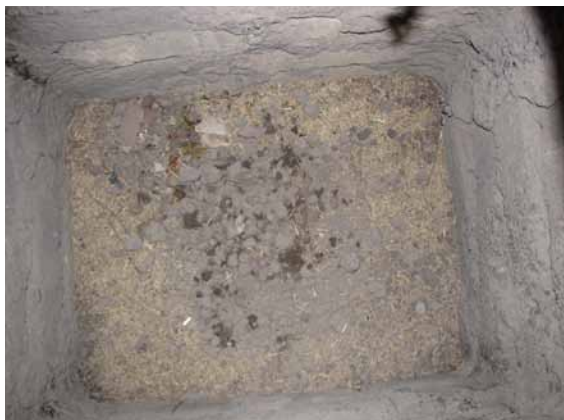
154 Inside of the granary space. LN 2010.
