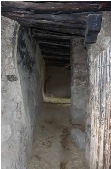
64 Passage to the tower room 12. HN 2010.
