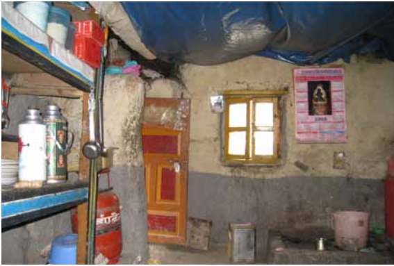
103 Southern outer wall of the staff quarters (29). DB 2010.
