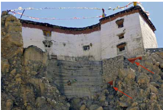
254 Underpin foundation elements along southern side of the ancient monastery. CA 2011.
