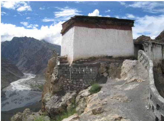
20 Retaining wall in the south-east of the upper temple. CA 2010.
