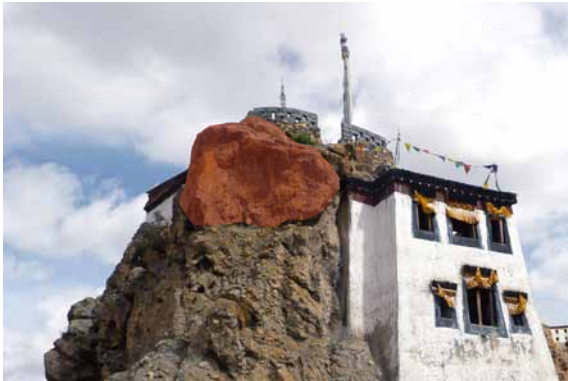
258 Support potentially unstable block along southern side of the tower. CA 2011.
