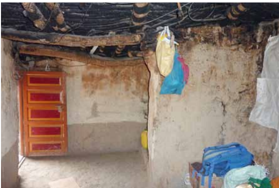
105 Room 30 with the access from the courtyard. HN 2010.
