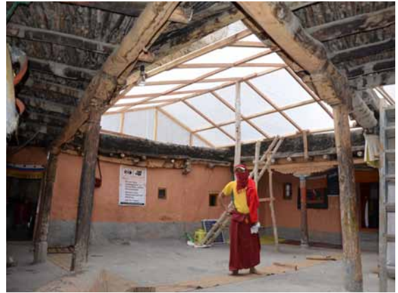
89 Temporary roof above the inner courtyard. CA 2011.
