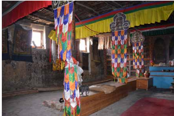
48 South-western part of the assembly hall. CA 2011.
