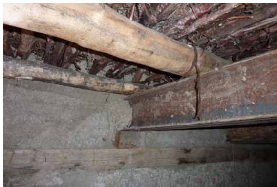
343 Detail of the new roof construction. HN2011.
