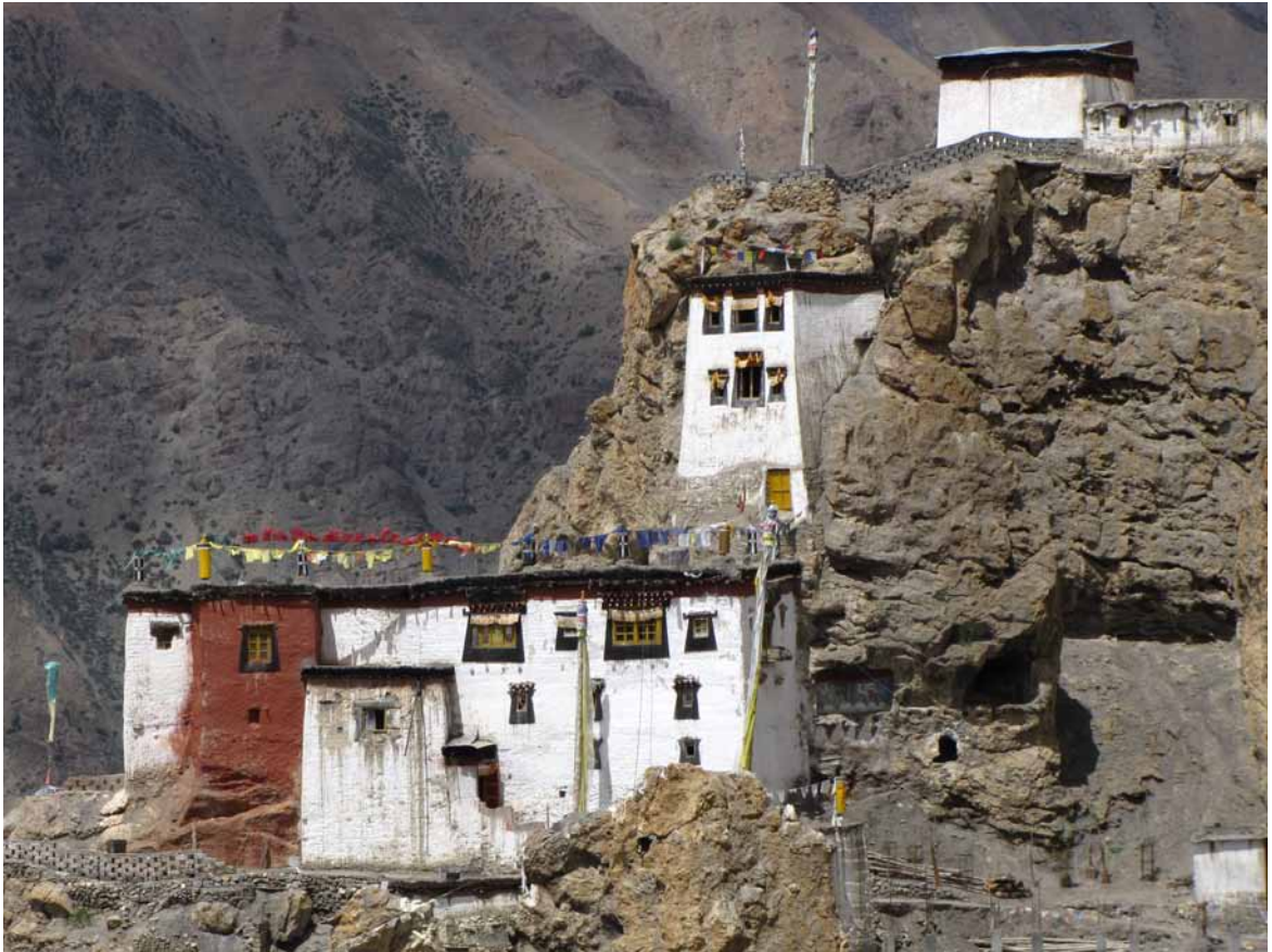
35 Eastern view of the monastery complex. LN 2010.
