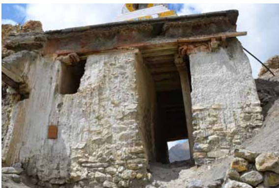
13 The north-eastern facade. CA 2011.
