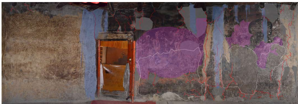
292 Map of the assembly hall. The eastern wall showing voids, cracks, washouts and drips, flaking and thinned painted surfaces. University of Applied Arts Vienna 2011.
