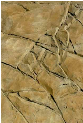
251 Example of textured and pigmented shotcrete wall. K&S 2011.
