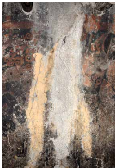
303 Repair-filling, deposits in form of channels. G&S 2011.
