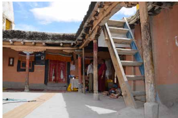
84 North and east side of the inner courtyard. CA 2011.
