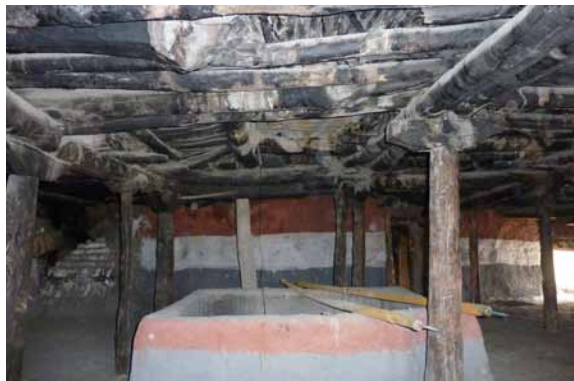
70 The former opening of the skylight in the middle area. HN 2010.
