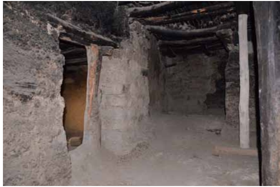
77 Room 19 with its entrance in the eastern wall. CA 2011.
