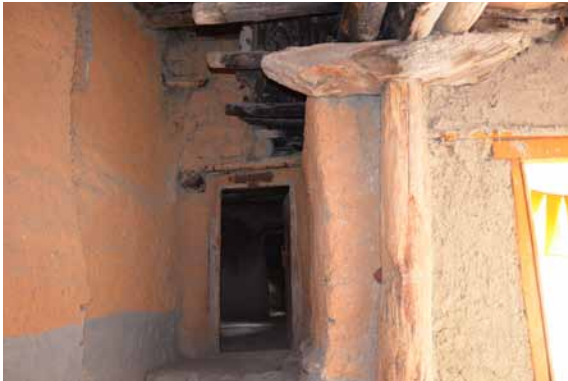
40 Access to the right side spaces of the entrance area. CA 2011.
