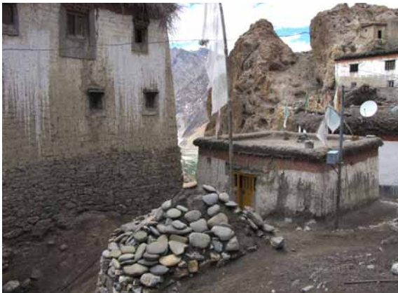
125 South-eastern view of the building. LN 2010.
