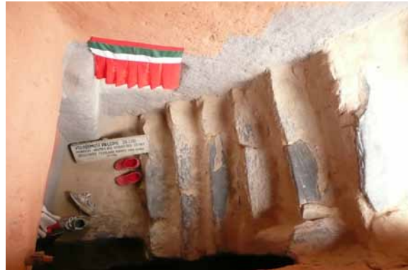
82 Stairway up to the third floor from above. CA 2010.
