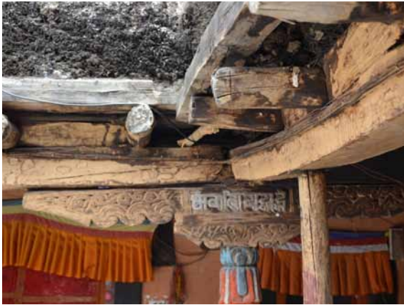
88 Corner detail of the wooden structure of the portico. CA 2011.
