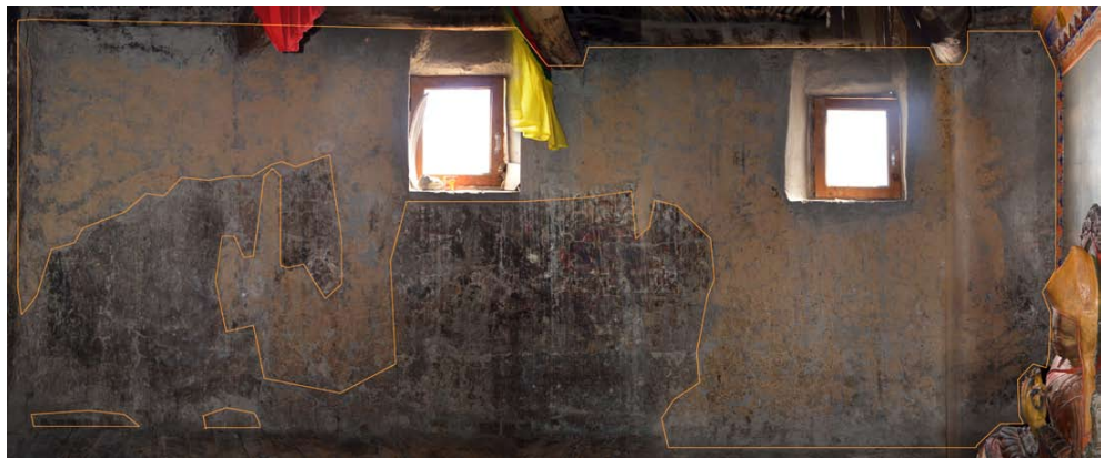
293 Map of the assembly hall. The southern wall with the extent of undecorated plaster, repair and recoated surfaces indicated. University of Applied Arts Vienna 2011.
