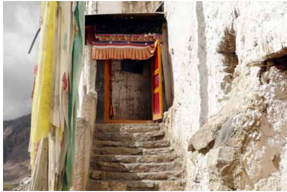
37 External staircase and entrance door to the main building. CA 2010.
