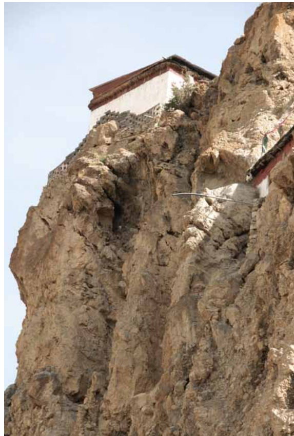
245 Condition of bimrock cliff along southern side of the upper temple. K&S 2011.
