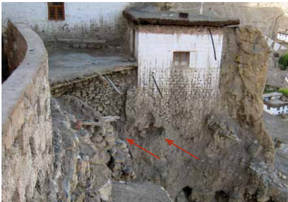
239 Partial undermining of block/mortar slope repair and foundation along southern side of the kitchen (note drain pipes). K&S 2011.
