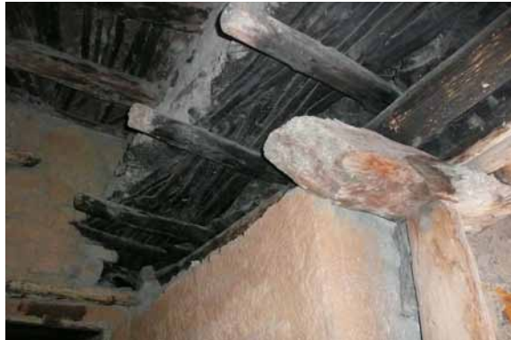
41 Cover construction of the corridor to the side rooms. CA 2011.
