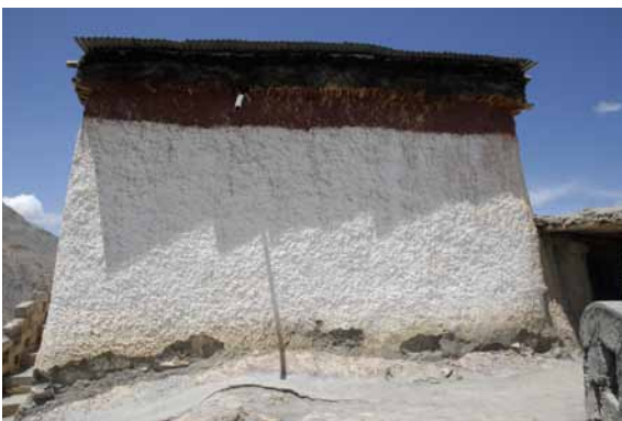
286 Outbreaks in the bottom zone of the upper temple. CA 2011.
