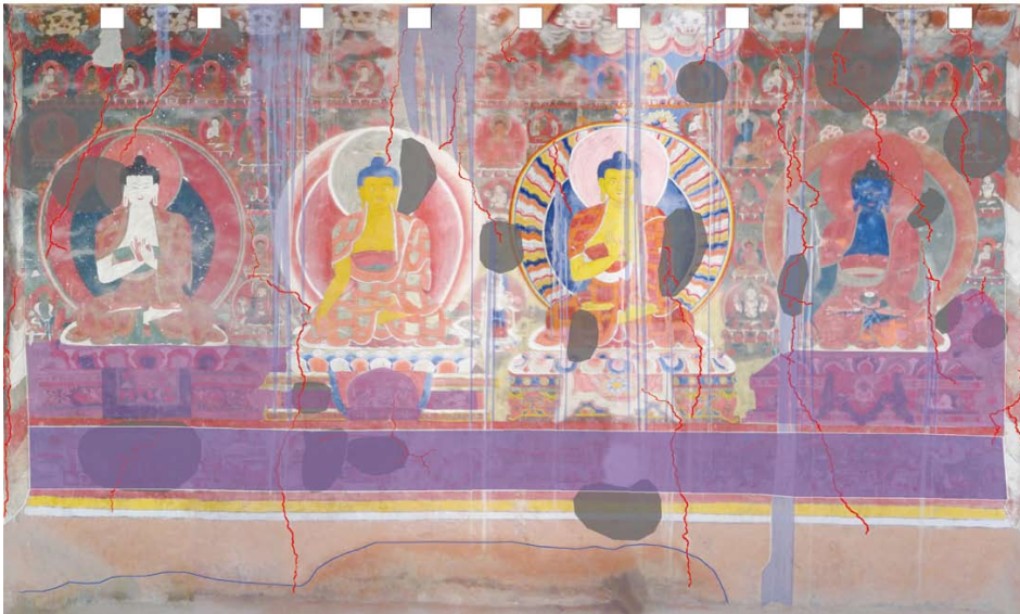
314 Map of the upper temple. The south-east wall showing voids, cracks, washouts and drips, a water horizon, flaking and thinned painted surfaces. University of Applied Arts Vienna 2011.
