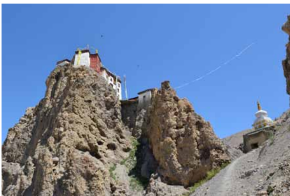
09 View of the building complex from the foot of the rock. CA 2011.
