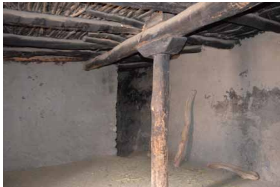
61 Northern and eastern wall with the entrance to room 12. CA 2011.
