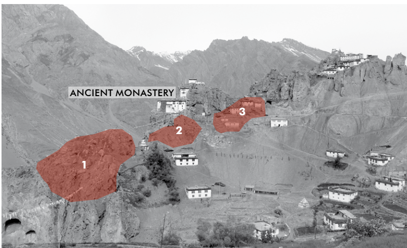
206 Condition of the existing ancient monastery, showing approximate areas of prior significant structures as indicated by historical portrayals. K&S 2011.
