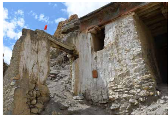
159 The window at the north-eastern facade. CA 2011.
