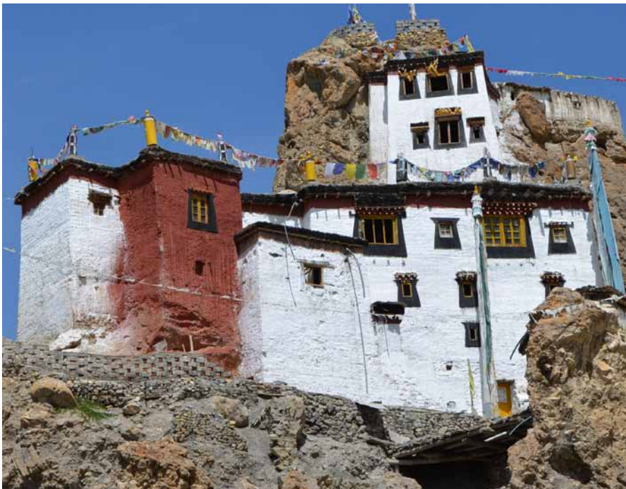
31 The east facade with the tower above the roof. CA 2011.
