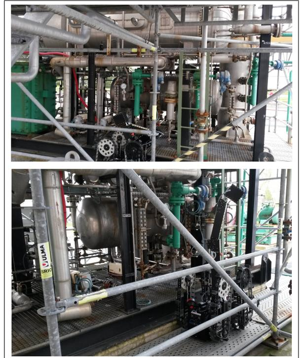
Fig. 1. Mobile robot approaching the liquid level gauge and positioning its arm to take a picture for level detection using image processing.
