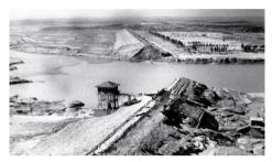
Figure 3. Final breach of Banqiao reservoir dam
