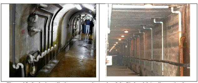
Figure 4 Left: drains relieving pressure in cracks of the Piedra del Aguila gravity dam (Hidroeléctrica Piedra del Águila, Argentina). Note goose necks on drains. Right: vertical drains in Platanovrissi RCC intercepting lift joints
