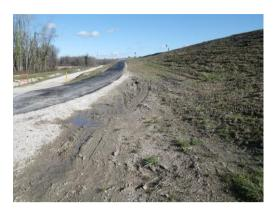
Figure 4: Picture of the draining ditch being excavated during works in 2014 (left picture), observation of humid soil (right picture).
