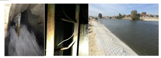
Figure 5. From left to right, joint 4-5 at Olai dam before and after underwater installation of Carpi external waterstop, and SIBELONMAT® installed underwater at Ismailia canal, Egypt 2016
