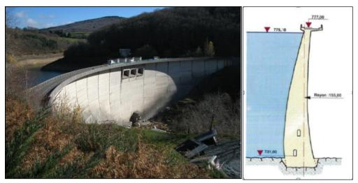
Figure 1. downstream view of the Laouzas dam and central cantilever design.
