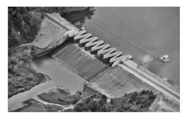
Figure 1: Example of a labyrinth weir (after Crookston and Tullis, 2013)
