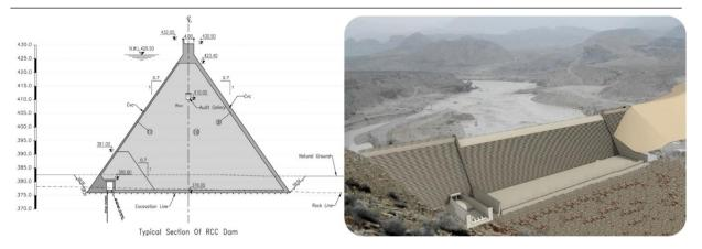
Figure 7. Dasht-e-Palang Dam (a combination of CMD & Earthfill)
