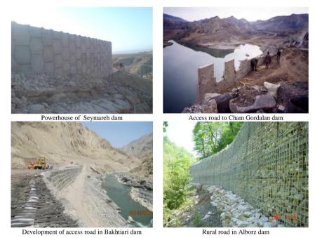
Figure 1. Pictures of reinforced soil walls in Iran dam projects
