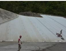
Figure 3. At left, Morávka dam at wintertime. At right, duckbill anchors being driven into the granular subgrade at Vaité earthfill dam
