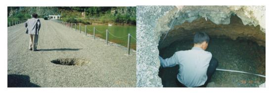
Figure 5. A sinkhole as a consequence of ageing that developed on the crest of the Unmun dam in 1998
