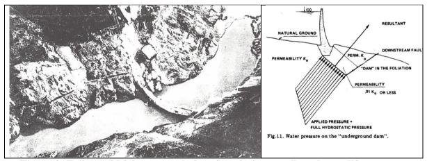
Figure 2: Failure of Malpasset arch dam foundation, attributed to uplift pressure (Londe, 1987)
