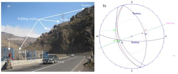
Fig. 5: a) A field photograph of right abutment dam showing the falling rock at the four locations toward the dam and road (view toward the northwest) and b) A stereonet showing the main sets, friction angle, and slope face plotted in dips V.5.1
