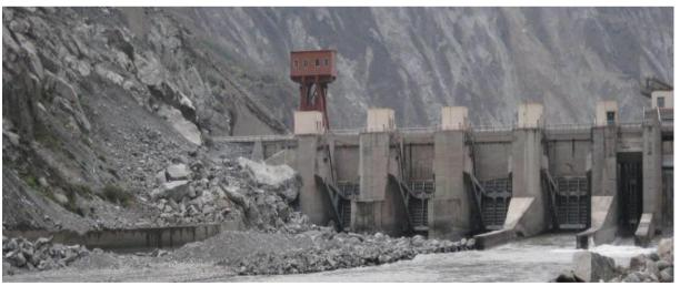
Figure 3: Damage of spillway piers caused by rockslides during the 2008 Wenchuan earthquake in China
