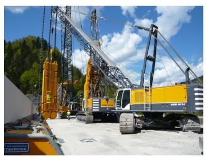
Figure 3. Cut-off wall equipment on a limited working platform
