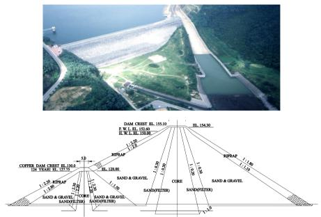
Figure 4. The Unmun dam before the sinkholes and excessive leakage accidents in 1998
