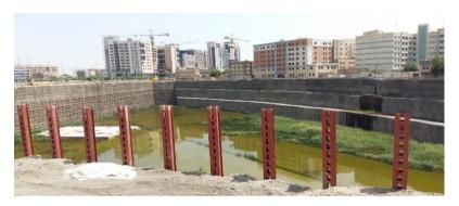
Figure 3. Water entering the construction sites.
