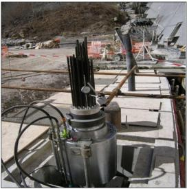
Figure 6 view of the downstream beam and of the installation of the anchors.
