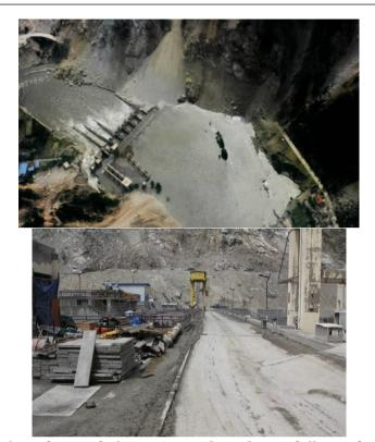
Figure 1. Overtopping of run-of-river power plant due to failure of gate operation (left) and mud deposited on crest of overtopped run-of-river power plant (right) (Wenchuan earthquake in China)
