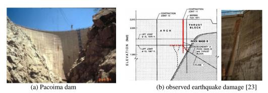
Figure 4. Observed damage of Pacoima dam in the Northridge earthquake
