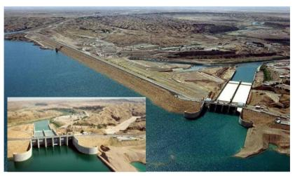
Figure 1- An example of the use of gated spillways with radial gates as a flood discharge system at the sideway of Karkheh dam in Khuzestan province in Iran.
