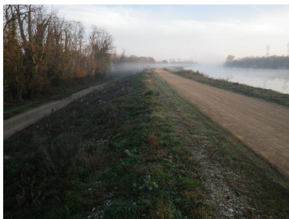
Figure 1: View of the canal embankment
