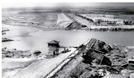
Figure 3. Final breach of Banqiao reservoir dam
