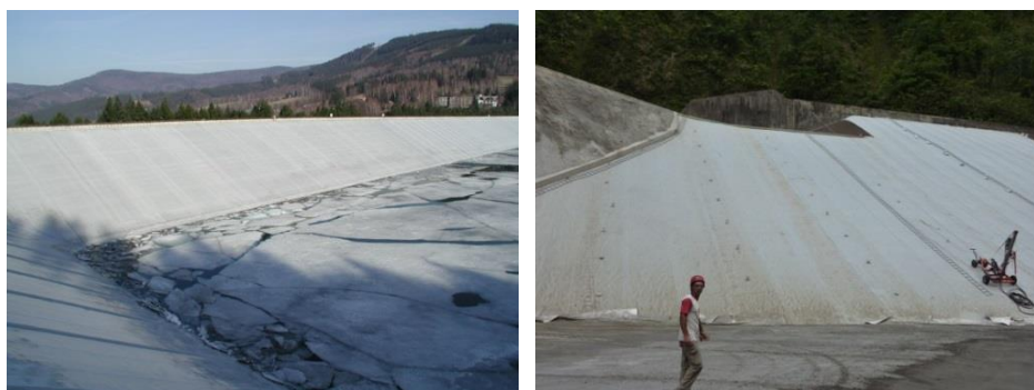
Figure 3. At left, Morávka dam at wintertime. At right, duckbill anchors being driven into the granular subgrade at Vaité earthfill dam
