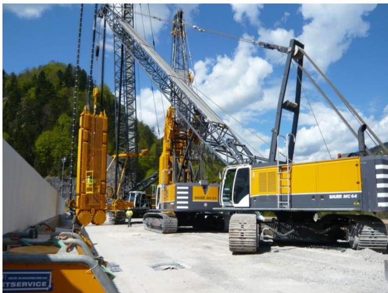
Figure 3. Cut-off wall equipment on a limited working platform
