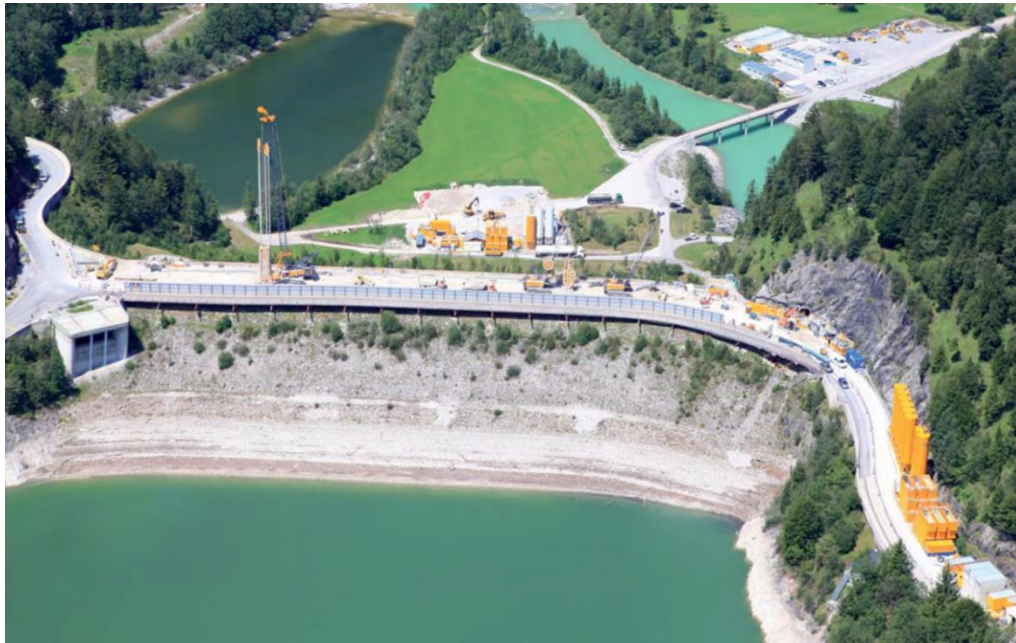
Figure 4. Cut-off wall installations with diaphragm wall grab, cutter and plants
