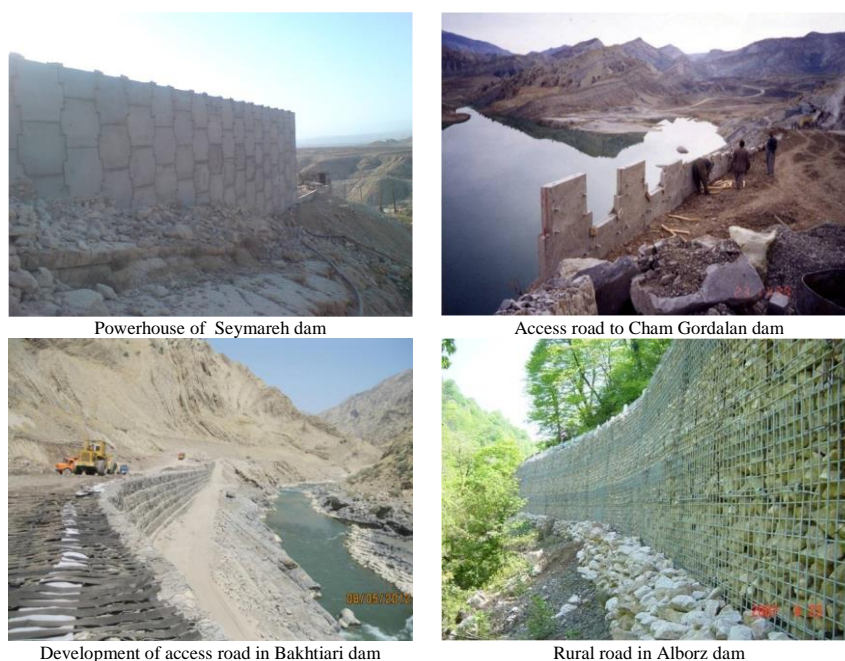
Figure 1. Pictures of reinforced soil walls in Iran dam projects
