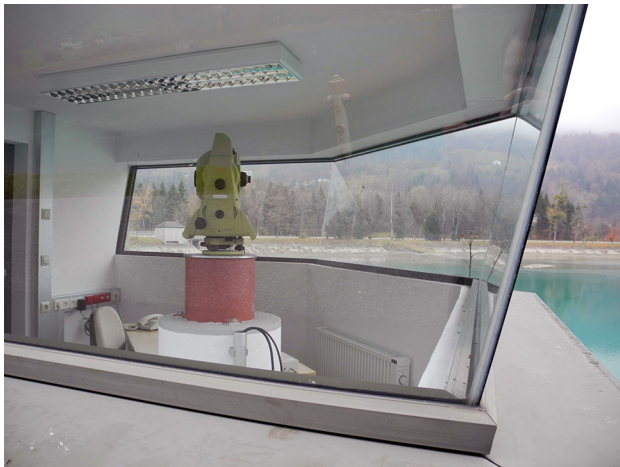
Fig. 2 RTS measurement setup for the monitoring of a water dam
