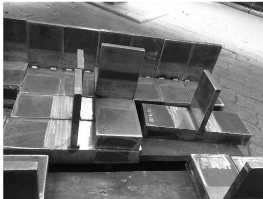
Fig. 1 Tack welded T-joints before welding.
