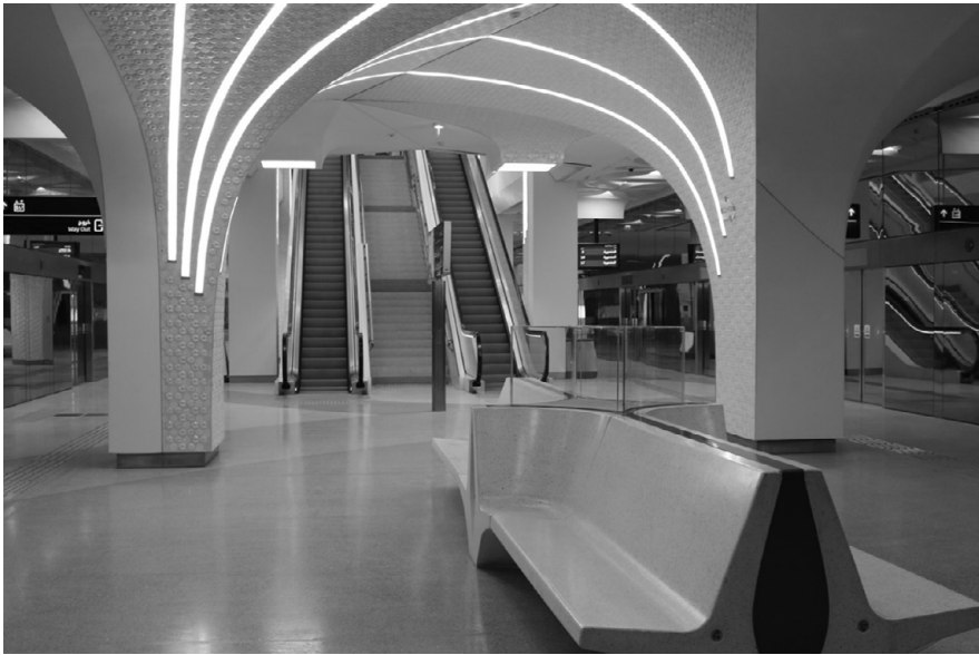
Fig. 14: Finishing Platform Level
