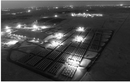
Fig. 7: Segment Production Facility
