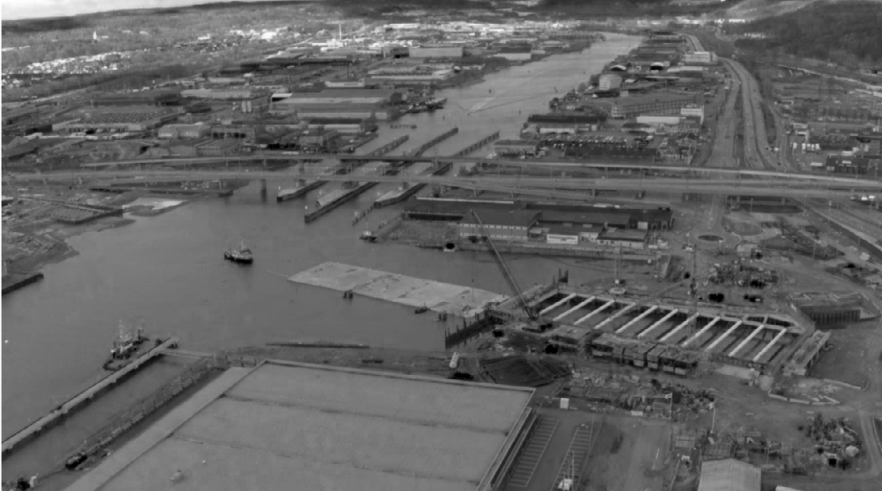
Abb. 10: Tunnelement 1 in Parkposition
