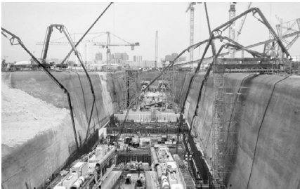
Fig. 11: Greenline Construction Pit Station
