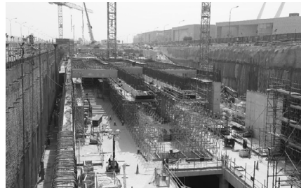
Fig. 12: Civil Works Al-Qadeem
