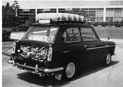
Fig.8. AFC powered Austin A40 hybrid city car of Prof. K. Kordesch [9]
