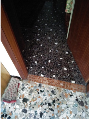
Fig. 3: Traditional solutions of reusing materials, residuals, as in the Venetian Terrazzo floor
