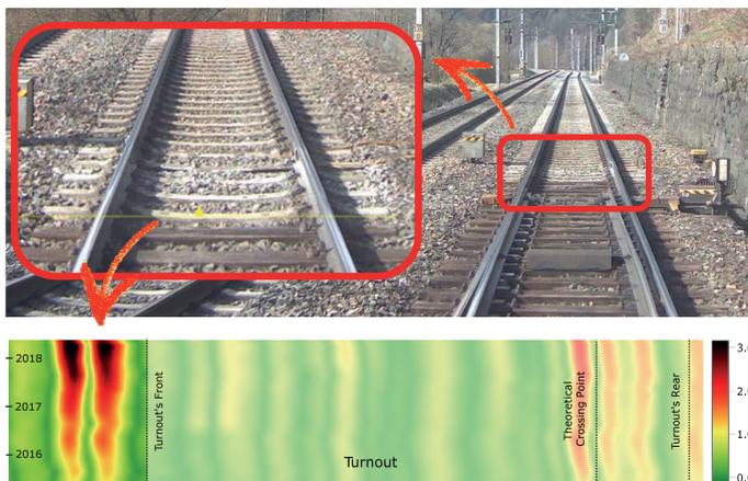
Figure 42 Example of insulated rail joint wear and ballast destruction.
