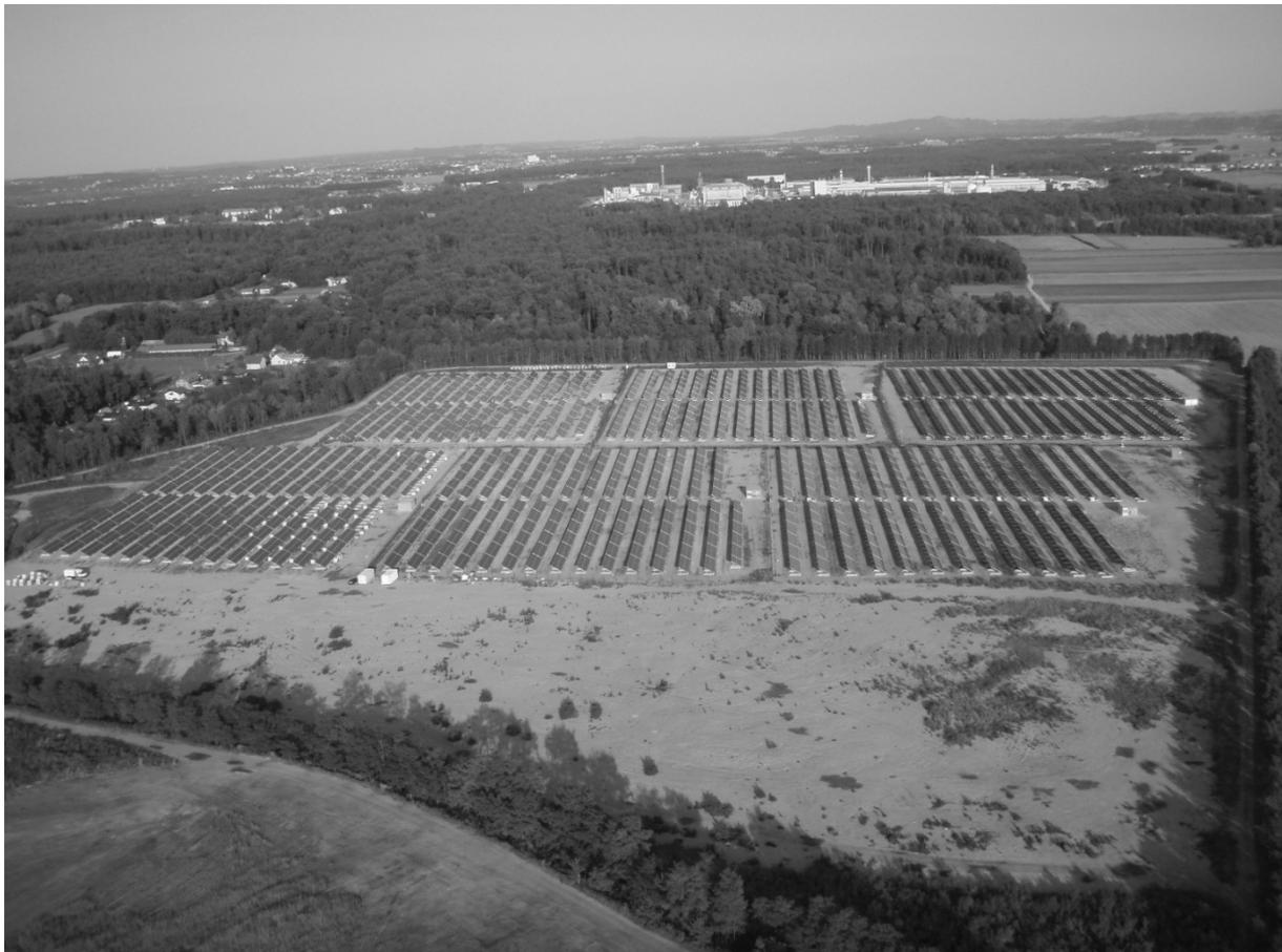
**Figure 1:** Solar field near Kidričevo (biggest in Slovenia) installed 6MWp on cca. 11 ha area
