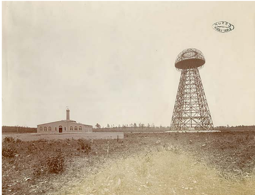
Fig.: Laboratory and Wardencllyffe Tower (Wikimedia Commons).
