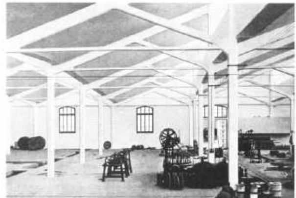
The seemingly zigzagging structure and the horizontal ties provide visual layers that mask the otherwise monumental sawtooth roof, domesticating the scale of the production hall
