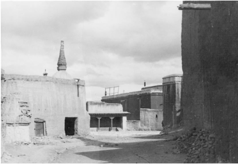
Fig. 29 West view of the Red Temple. In the front, you can see the northern façades of the Main Temple. Tucci expedition, E. Ghersi 1933. ©_Museo delle Civiltà – MAO G. Tucci.
