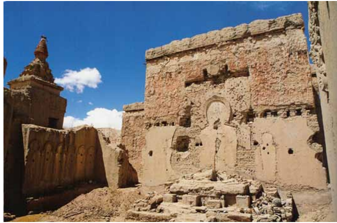
Fig. 44 The assembly hall of the Main Temple after the excavation of the original floor level before the restoration. On the rear wall, halos and beam holes allow clear conclusions to be drawn about the size of the main figure and the height of the lantern and ceiling construction. Zong Tong-Chang, in NAMGYAL 2001: 78.
