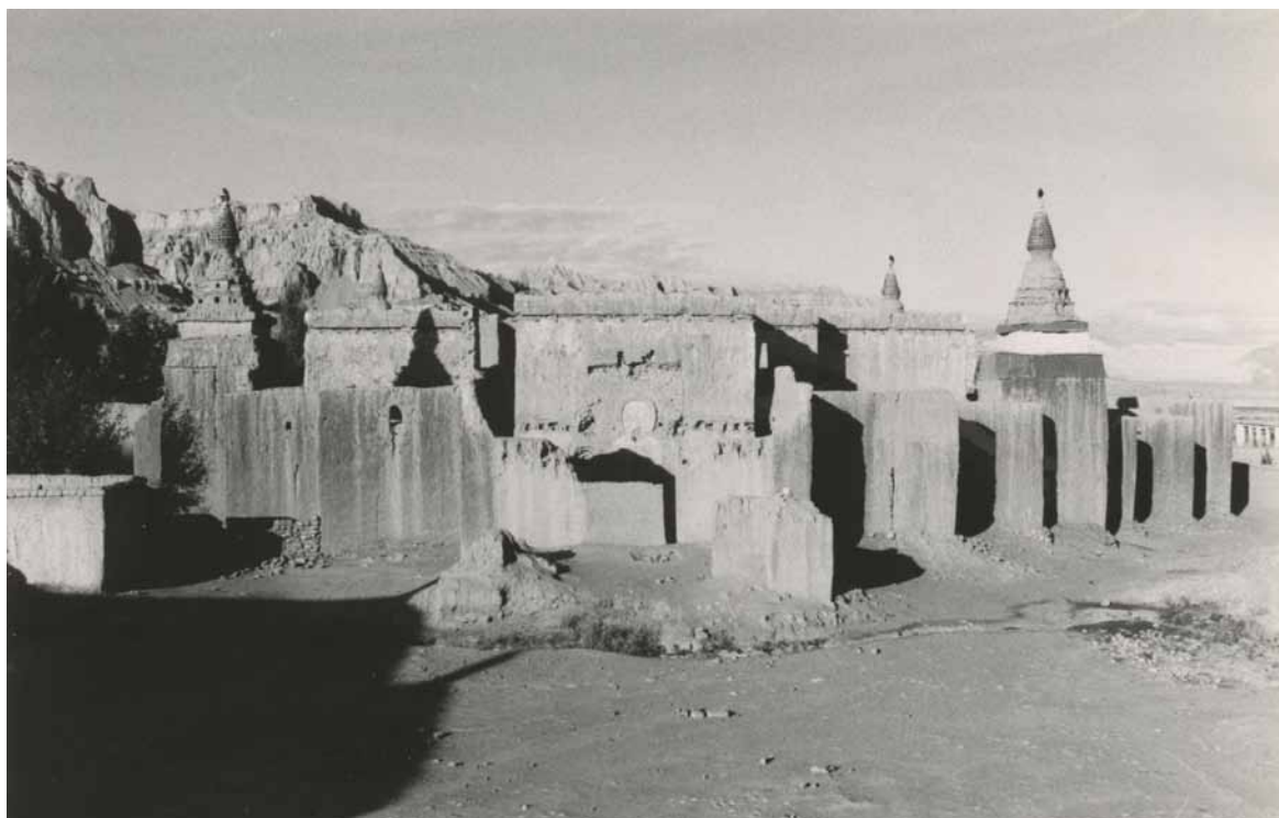
Fig. 52 Northeast view of the Main Temple with the fragments of the assembly hall and the vestibule. The beam holes in the wall show traces of the construction above the vestibule. Luczanits 1993.
