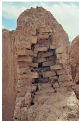
Fig. 564 Left. The outer layers of the brick masonry of the temple ruins of Basgo show an orderly brick bond, while the interior shows the dissolved state of the bond. Neuwirth 2004.
