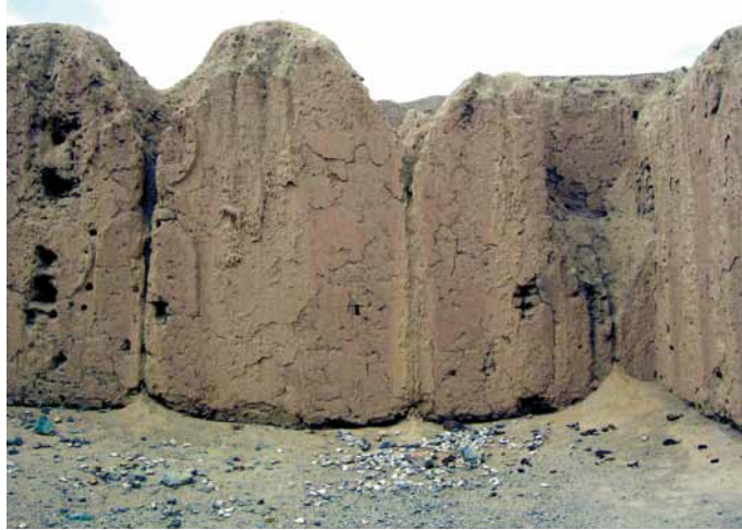
Fig. 465 East part of the north wall inside the main room of the ruin. Luczanits 2009.
