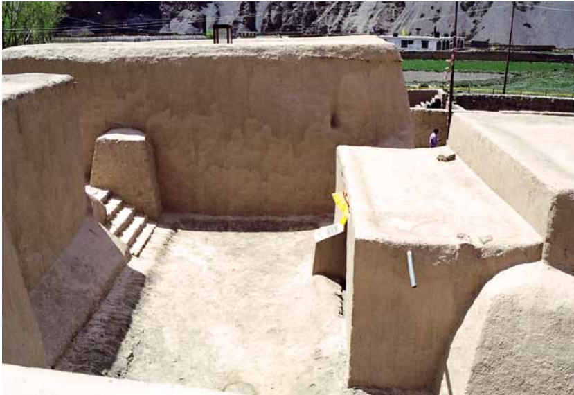
Fig. 332 The forecourt in front of the Mandala Temple is formed by the north façade of the Golden Temple and the west façade of the Large 'Bromston Temple. Auer 2003.
