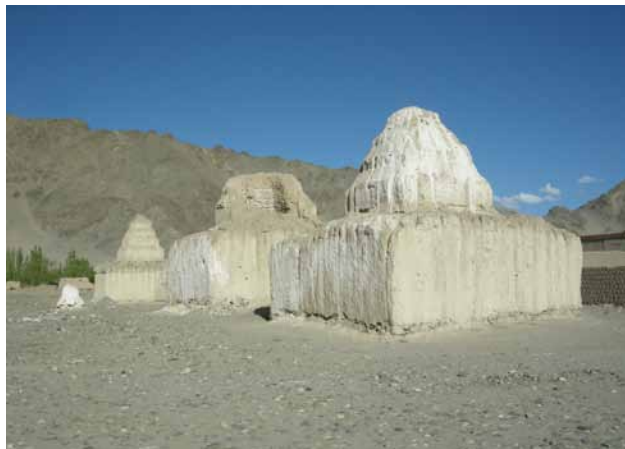
Fig. 201 Three huge chörten standing on the south side of the area, directly in front of the still-existing fragments of the surrounding wall. The side lengths are between 6.50 metres and 7.70 metres, the height of the base is 3.40 metres on average and about 6 metres at most. Luczanits 2009.
