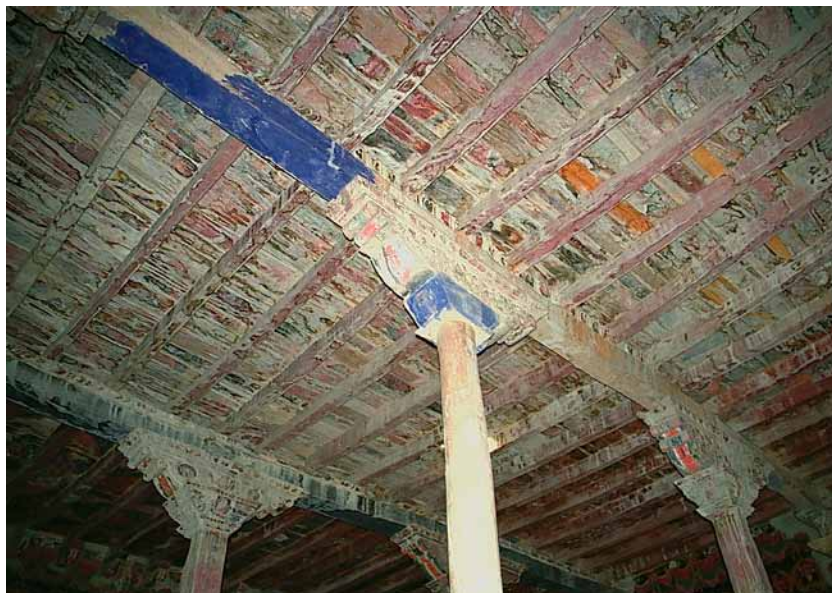
Fig. 316 The two main beams of the ceiling construction facing northwest. Neuwirth 2002.
