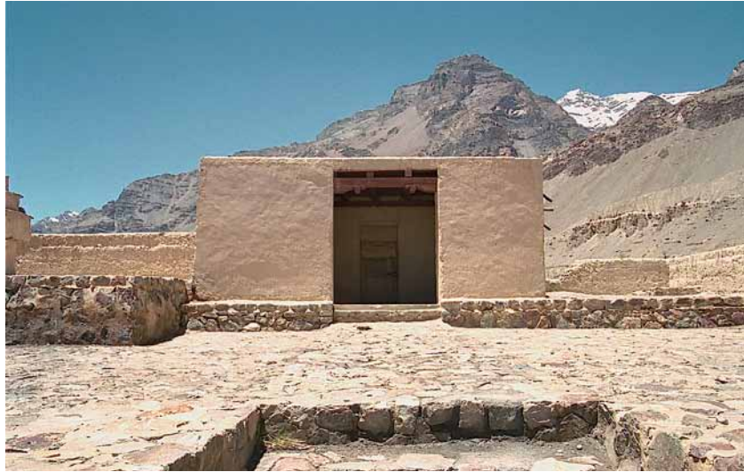
Fig. 354 Eastern view of the White Temple with the vestibule, which was not set up until the renovation. The surrounding walls of the monastery are directly connected to the side walls of the main room. Neuwirth 2002.
