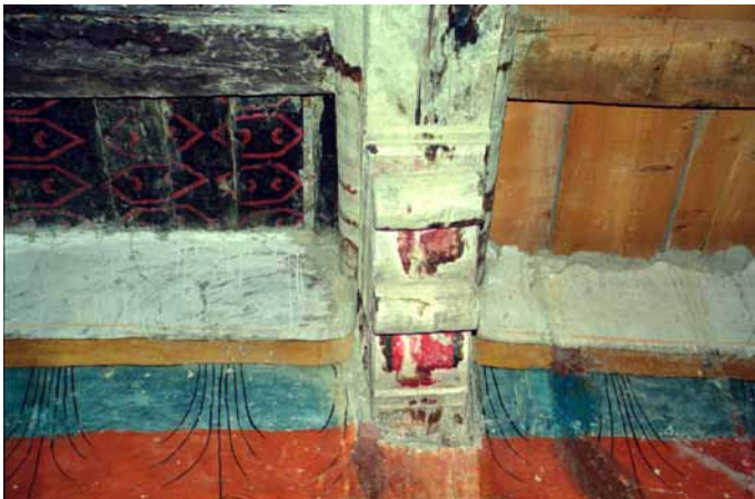
Fig. 415 Wall console on the north wall, with the remains of the ceiling painting, and the partially renewed sections. Neuwirth 2002.
