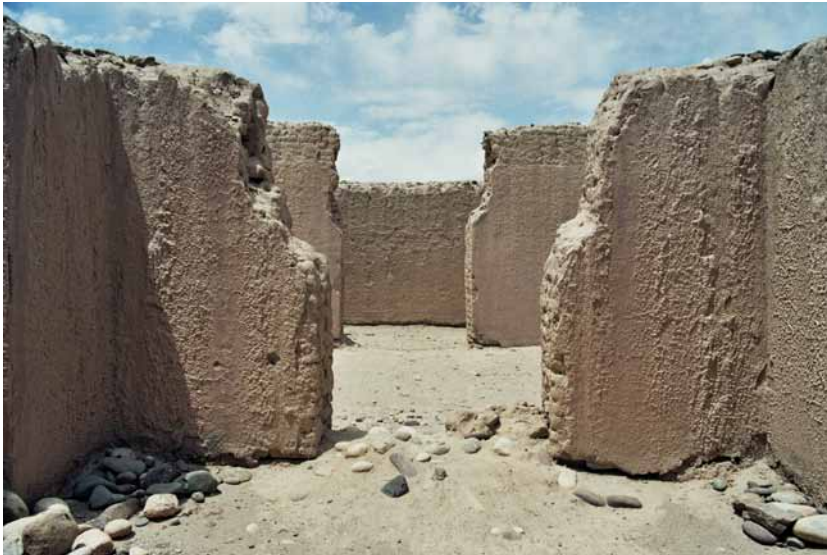
Fig. 190 Line of sight from the interior of Temple No. 4 to Temple No. 3. Above: the still relatively well-defined entrance openings, whereby the wall breakouts extend from the point where the door lintels were once positioned. Auer 2004.
