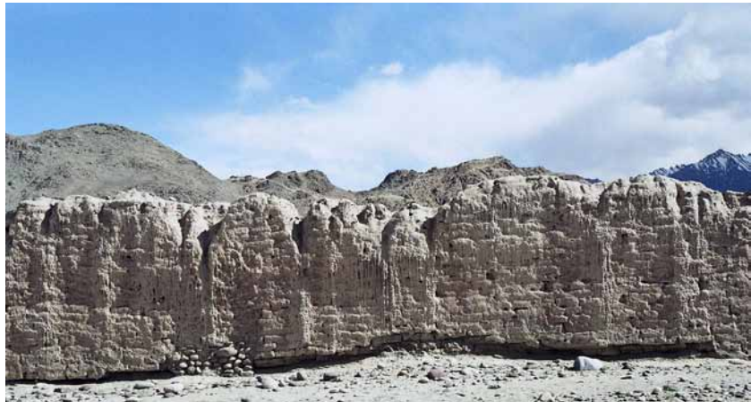
Fig. 487 The remains of the surrounding wall of Nyarma's sacred compound. The wall fragments in various lengths are 0.60 to 0.80 metre thick and between 1.20 and 2.90 metres high. The upper edge and bottom zone of the homogeneous brick wall have been strongly eroded by weathering, but some plaster layers are still visible. Neuwirth 2003.
