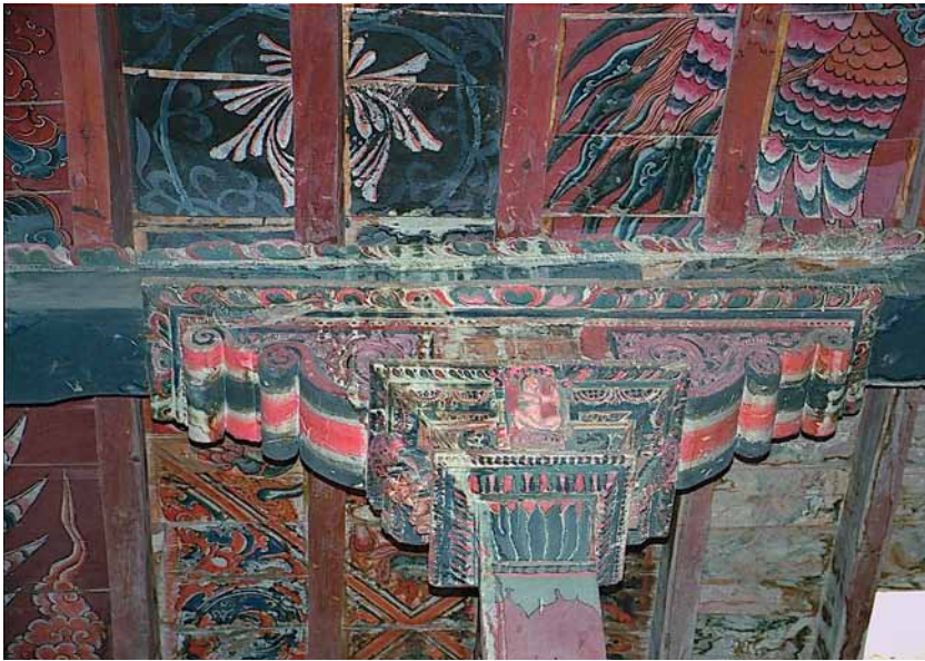
Fig. 314 West side of the carved and coloured console capital above the northwest support of the ceiling construction. Neuwirth 2002.
