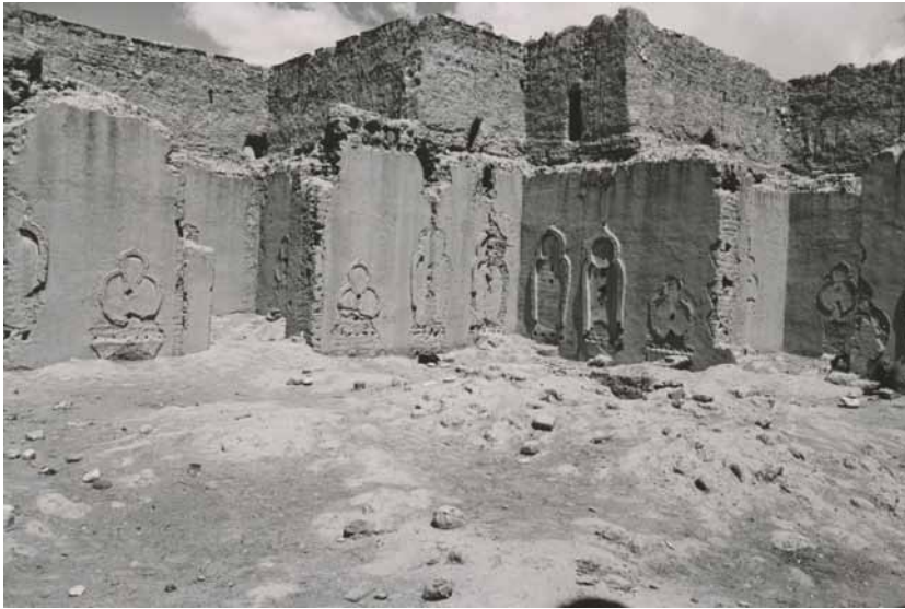
Fig. 53 The central room of the Main Temple with the entrance in two of the four main chapels. The different wall surfaces and the beam holes show the previous construction of the ceilings. The floor was buried up to one metre high before it was uncovered. Luczanits 1993.
