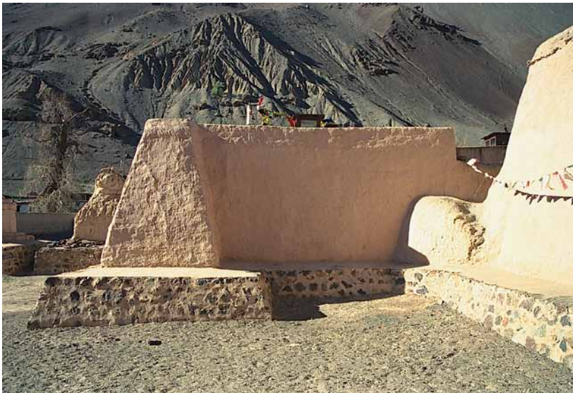
Fig. 333 South view of the Mandala Temple with the projecting abutment on the west side of the temple and the surrounding base zone made of stone masonry. Neuwirth 2002.
