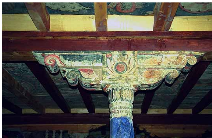
Fig. 286 Above: two Examples of the coloured console capitals in the assembly hall of the Large 'Brom-ston Temple, supporting the main beam of the ceiling construction. Below: one of the coloured wall consoles is shown on the side walls of the assembly hall. Neuwirth 2002.
