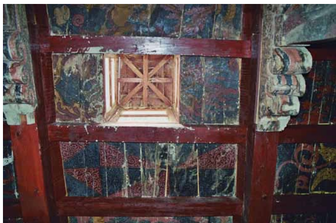
Fig. 343 Skylight of the lantern in the central area of the painted ceiling. Neuwirth 2003.
