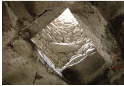
Fig. 207 View upwards into the corbel vault of the chörten, which is made of mudbricks in the upper part and round river stones in the lower part. Luczanits 2009
