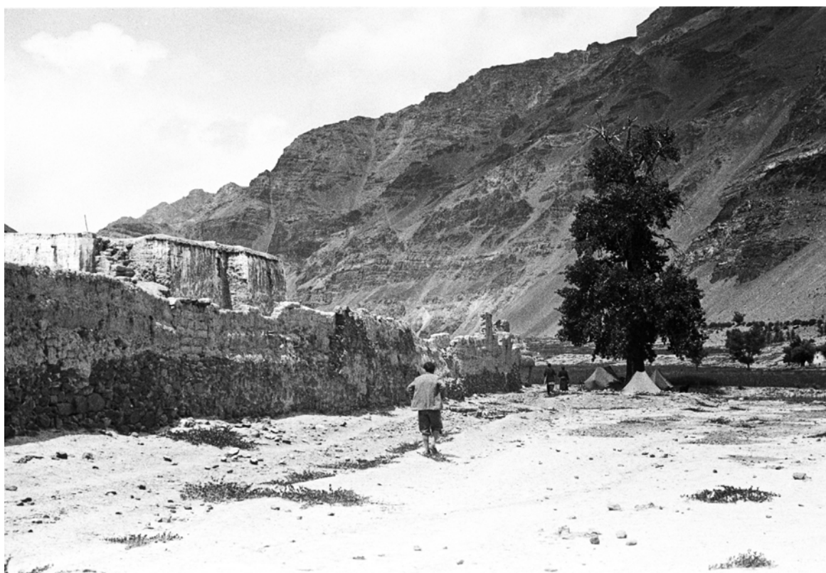
Fig. 225 North side of the enclosing wall with the upper part of the Small 'Brom-ston Temple inside the compound. Tucci expedition, E. Gherzi 1933. ©_Museo delle Civiltà – MAO G. Tucci.
