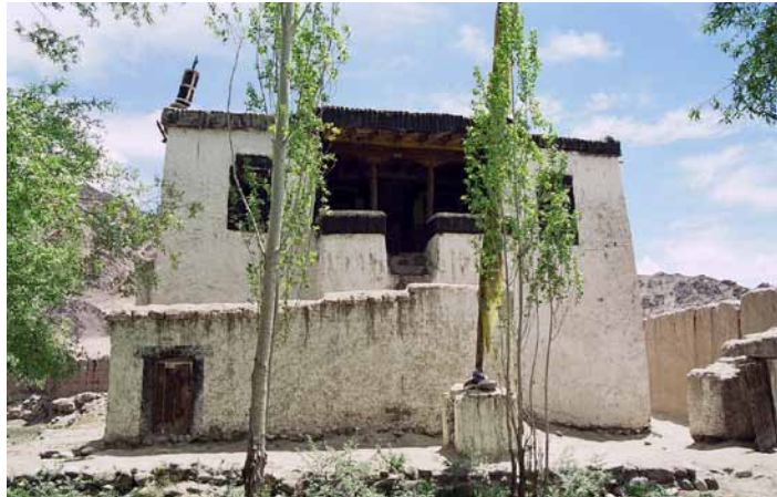
Fig. 169 View of the Main Temple from the west with the entrance to the ground floor as well as to the Dorje Chenmo Temple on the first floor. Neuwirth 2003.
