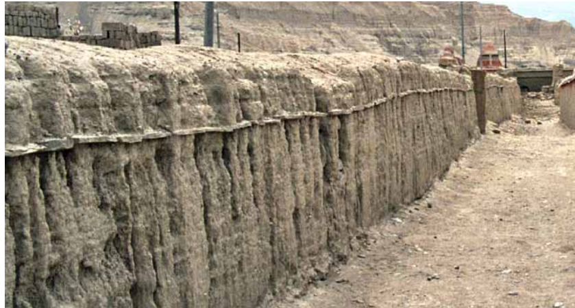
Fig. 489 The construction of the southeast surrounding wall of Tholing. The lower part is made of rammed earth, and a layer of clay bricks is found above a thin layer of stone slabs, which indicates a weathered row of chörten. Neuwirth 2007.
