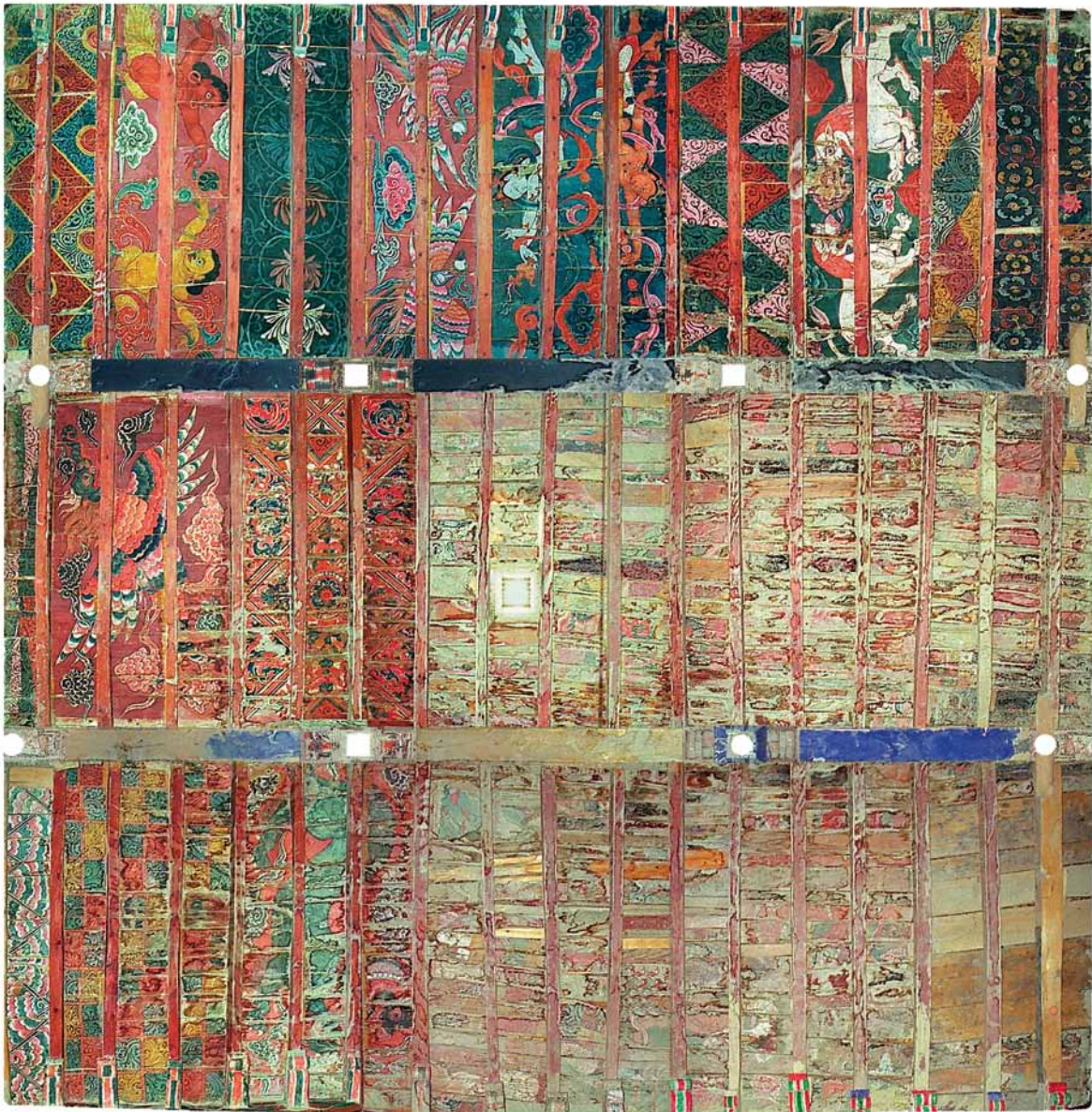
Fig. 318 Scaled photomontage of the painted ceiling in the Golden Temple. The painting in the third yoke in front of the west wall shows the best state of preservation. © Neuwirth & Auer, TU Graz 2020.
