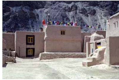
Fig. 236 Left: Southern view of the east building with the former monastery kitchen on the ground floor and residential rooms on the upper floor. Neuwirth 2003.
