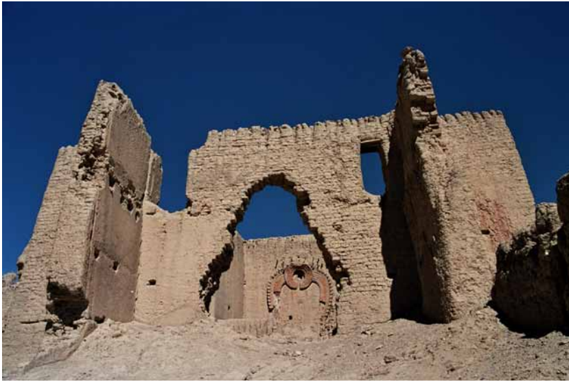
Fig. 132 The entrance to the main room of the temple ruin with the wall openings and the row of beam holes in the former ceiling. Neuwirth 2007.
