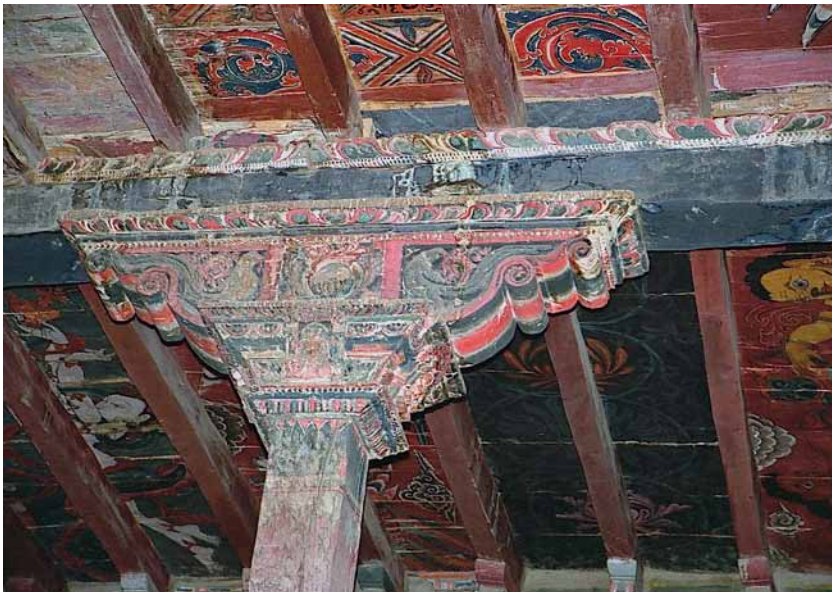
Fig. 315 East side of the carved and coloured console capital above the northwest support of the ceiling construction. Neuwirth 2002.
