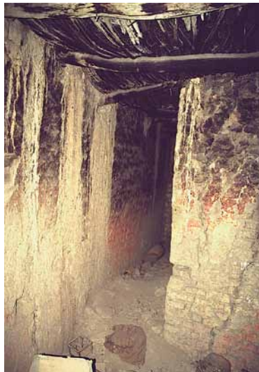
Fig. 277 The space between the outer walls of the Large 'Bromston and the Main Temple. The traces of the red wall painting in the lower part of the façades are still clearly visible. Left: the east walling in the back, which consists of a rammed clay wall. Right: the corner between the vestibule and the assembly hall of the Main Temple. The brick formats and a settlement crack are clearly visible in the lower area of this picture. Neuwirth 2002.
