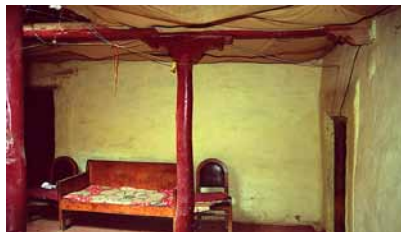
Fig. 273 Left: the entrance from the outside stairway to the lobby in the upper floor above the kitchen. Right: the entrance room with the accesses to the other rooms of the upper floor. Neuwirth 2002.
