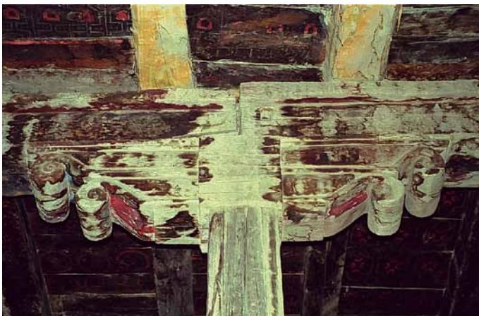
Fig. 416 Console capital under the main beam, with remains of the former colourful painting. Neuwirth 2002.
