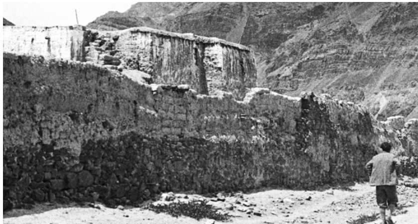
Fig. 488 The surrounding wall on the north side of Tabo's sacred compound shows a patchwork of different techniques and heights on the outside. Tucci expedition, E. Ghersi 1933. ©_Museo delle Civiltà – ©MAO G. Tucci.
