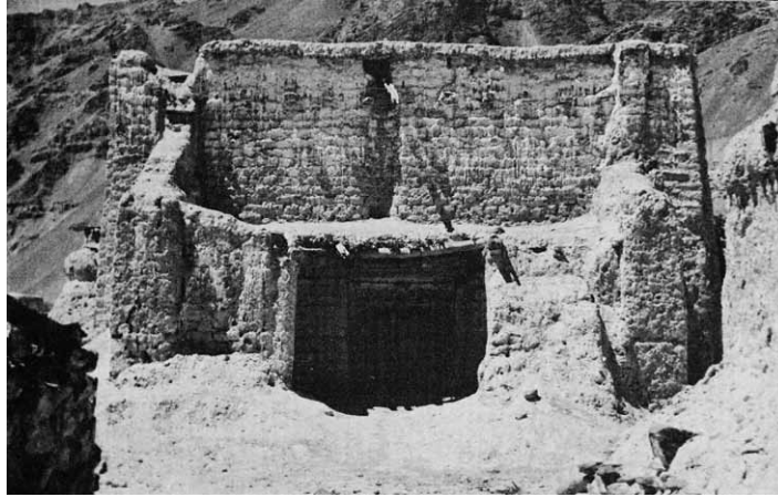
Fig. 593 The modifications and changes of the appearance at the eastern facade of the Maitreya Temple of Tabo. Khosla 1979, Illustration 44.
