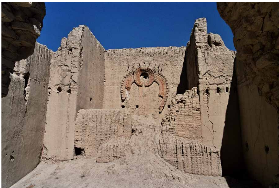
Fig. 137 The view from the vestibule into the main room with the apse located in the northwest. A brick wall was built directly adjacent to the corners of the apse, and separates the area from the main room today. Neuwirth 2007.
