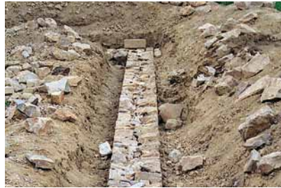
Fig. 553 Right: Foundation and lower zone of the exterior wall, made of quarried stones with clay mortar. Neuwirth 2002.
