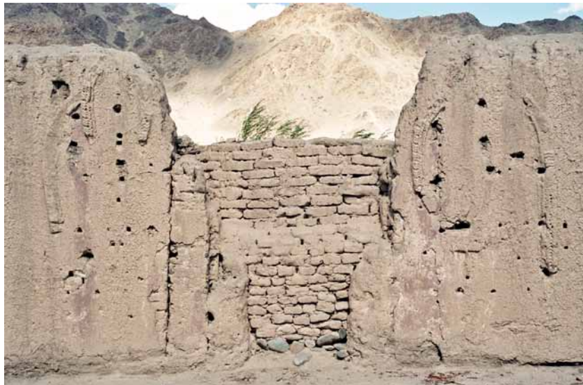
Fig. 166 The masonry on the east side of the assembly hall clearly shows the traces of the former opening. Vestiges of former halos and plug holes are preserved on both sides of the original entrance opening. Auer 2003.
