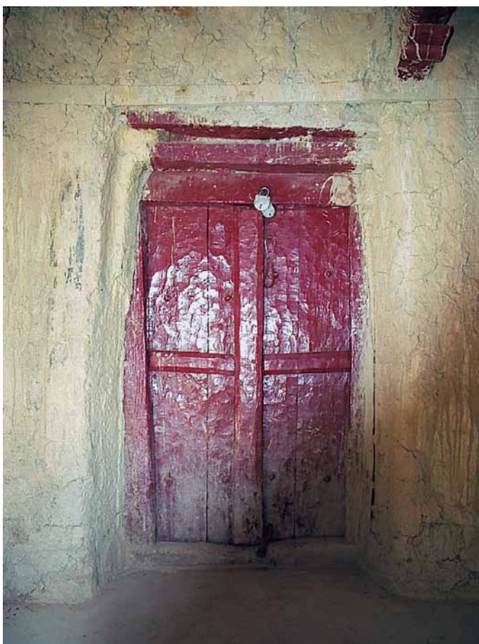
Fig. 449 The door on the northwest side of the entrance hall leads into the innermost chapel in the rear of the complex: Neuwirth 2002.
