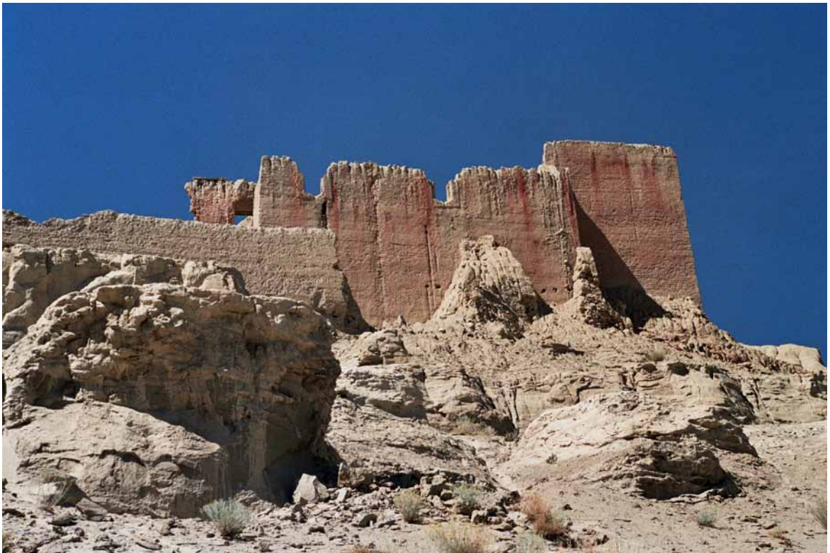
Fig. 133 North-eastern view of the temple's exterior walls with the height staggering of the different areas and the significantly higher apse. Neuwirth 2007.
