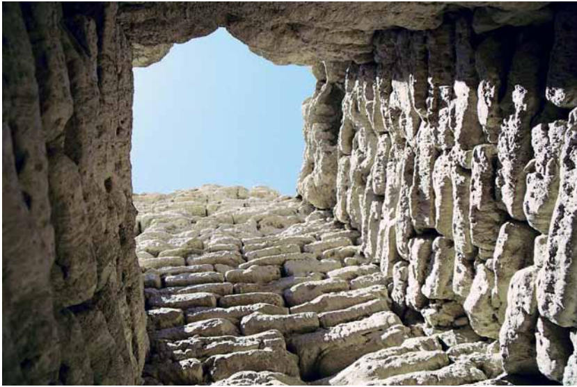
Fig. 198 The inner surfaces of the walls of the chambers, which are laterally connected to the apse walls, are non-plastered. Both chambers were originally inaccessible. Neuwirth 2003
