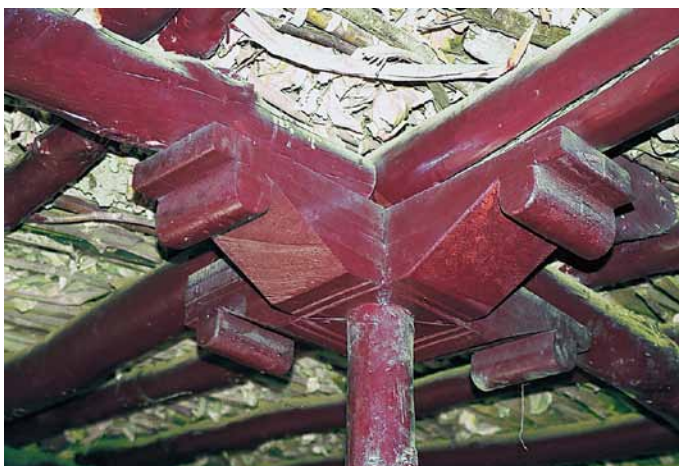
Fig. 448 One of the four cross- consoles of the ceiling construction in the entrance hall. Neuwirth 2002.
