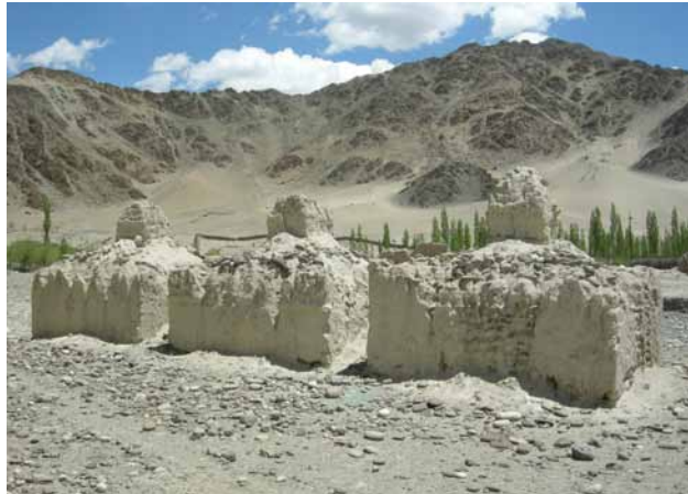
Fig. 200 A row of three weathered chörten on the east side of Temple No. 4 with side lengths between 2.70 and 2.80 metres. Due to the absence of the plaster layer, the underlying construction becomes visible. Luczanits 2009.
