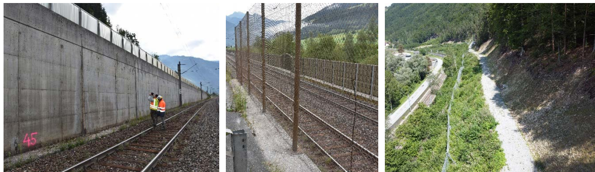
Figure 7: Example of assets along the Austria railway lines, retaining structures (left), noise-protection constructions (centre), natural hazard-protection structures (right)
