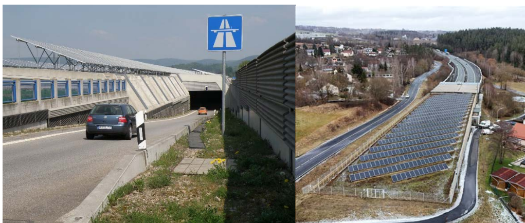
Figure 3: PV-modules on noise protection tunnels (photo: left: BASt, right: Autobahn GmbH, NL Nordbayern)
