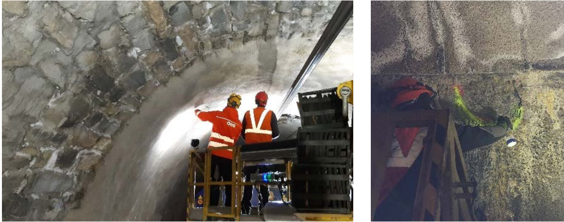
Figure 5: Inspection and documentation of the lining of a tunnel
