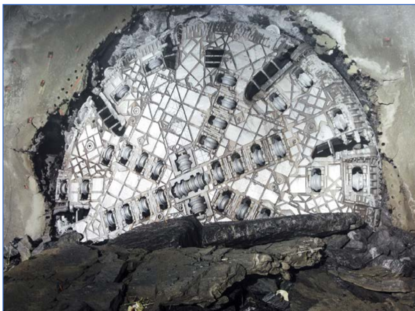
Figure 2: Koralm Tunnel – final breakthrough June 17, 2020
