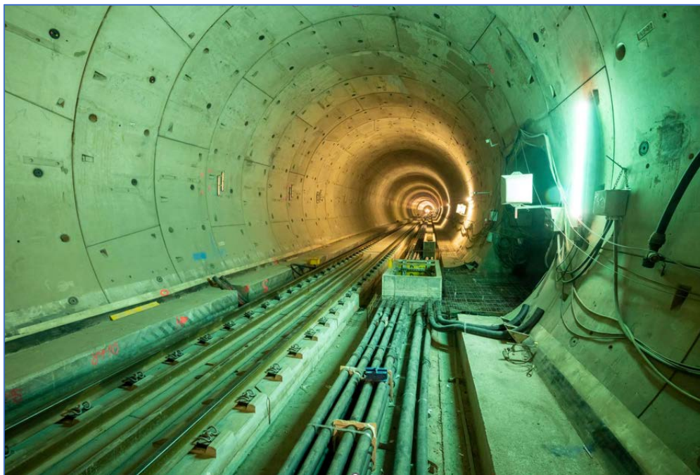
Figure 4: Koralm Tunnel – intermediate state of construction, December 2021
