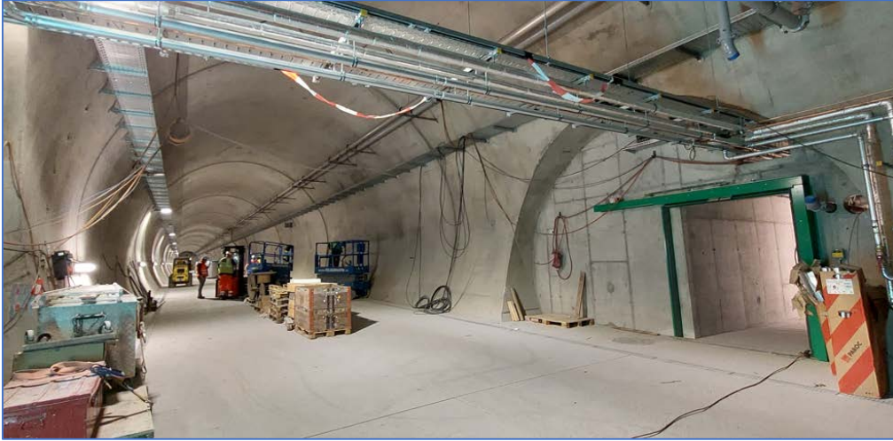
Figure 5: Koralm Tunnel emergency station – intermediate state of construction, January 2024
