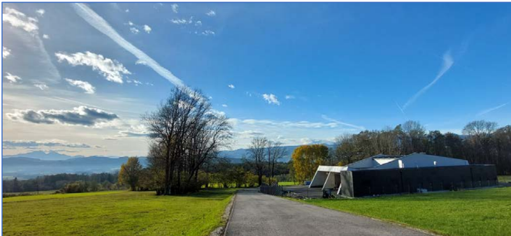
Figure 6: Koralm Tunnel – West Paierdorf ventilation building, November 2023
