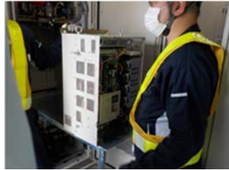
Figure 6: Exchanging the inverter unit
