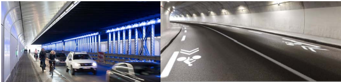
Figure 4: Road tunnel with mixed traffic (photo: left: Henning Koepke, right: CETU)
