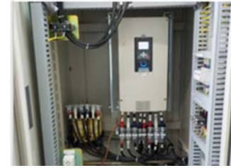
Figure 7: 2-level inverter unit installed in the control
