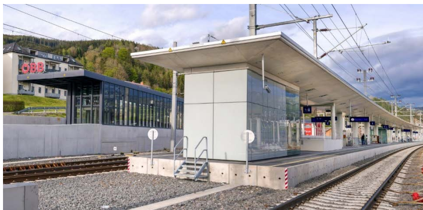
Figure 5: Station Mürrzuslag, platform 4/5
