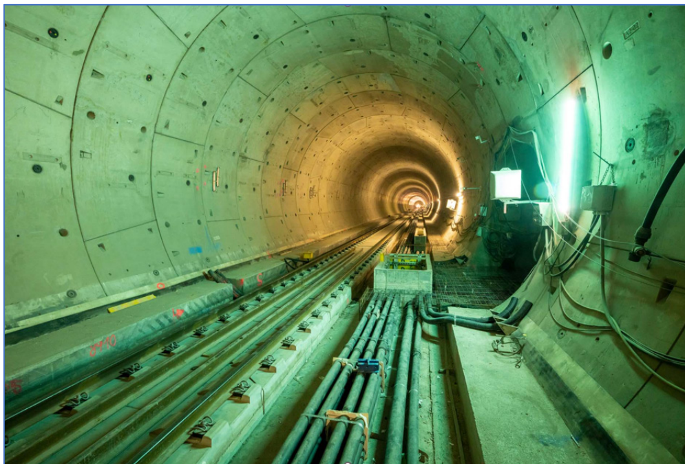
Figure 4: Koralm Tunnel – intermediate state of construction, December 2021
