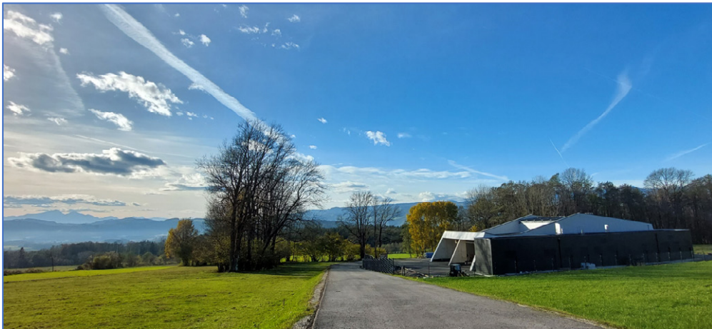
Figure 6: Koralm Tunnel – West Paierdorf ventilation building, November 2023
