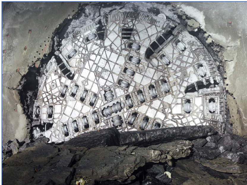
Figure 2: Koralm Tunnel – final breakthrough June 17, 2020
