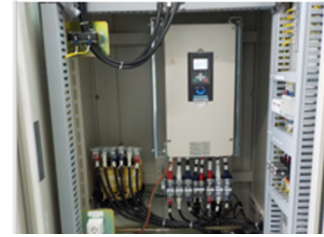
Figure 7: 2-level inverter unit installed in the control
