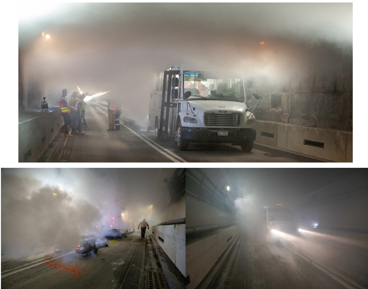
Figure 7: Images of the Delve Stacey Agnew Smoke Bus at various stages of different tests, producing copious quantities of hot ‘smoke’ in service of demonstrating visually the ventilation system performance.
