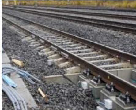
Figure 1. An overview of the test site including a transition zone between ballasted track and 3MB slab track at Gransjö, north of Boden, Sweden.
