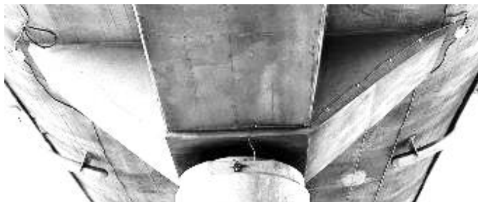
Figure 1. Sensors installed under the deck of viaducts over piazza Maggi.
