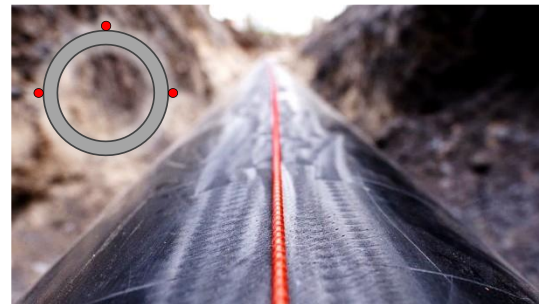
Figure 16. Distributed strain sensors (EpsilonRebars) during the installation (just before gluing) directly on the pipeline.
