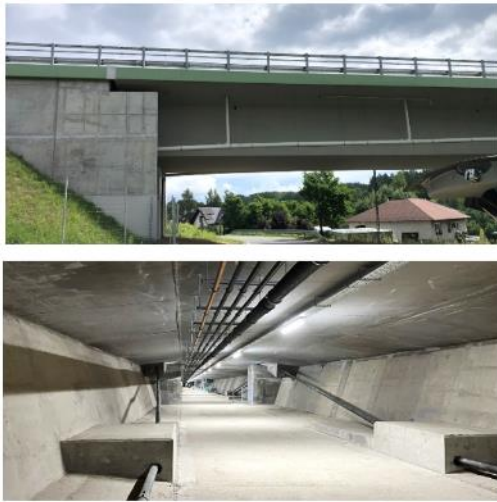
Figure 8. General view of the analysed bridge from the outside (top) and inside of the prestressed box (bottom).
