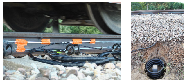
Figure 7. Connections between segments of the sensors during installation and the view of the protective well.
