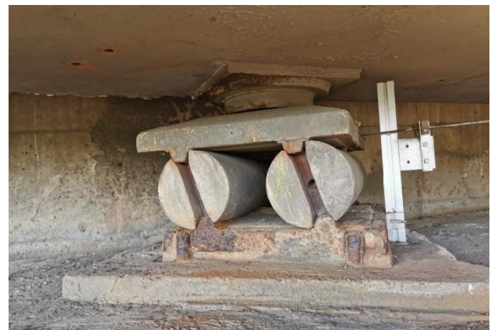
Figure 3. Monitoring system on the bridge bearing.
