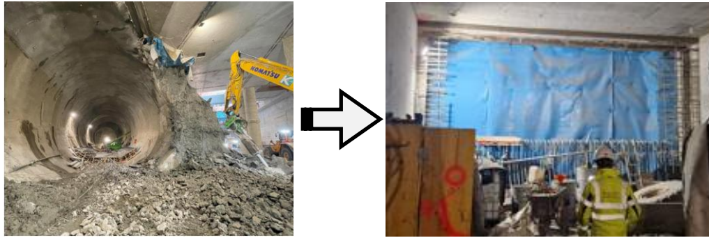
Figure 1 (Left) Recycled aggregates (RA) claimed from a demolished subway tunnel section and (Right) diaphragm wall section intended for applying recycled aggregate concrete (RAC)
